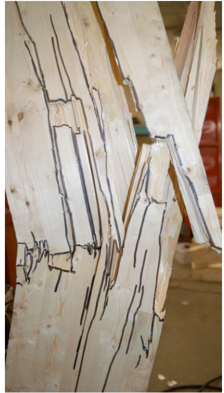
(c) Close-up of mid-span damage for C2.3-[137]
