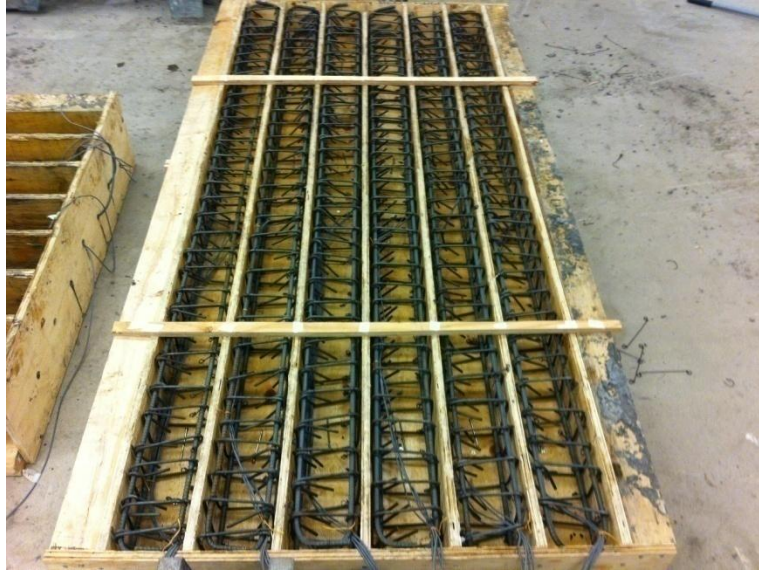
Figure 3.7 Formwork containing six complete specimen cages
