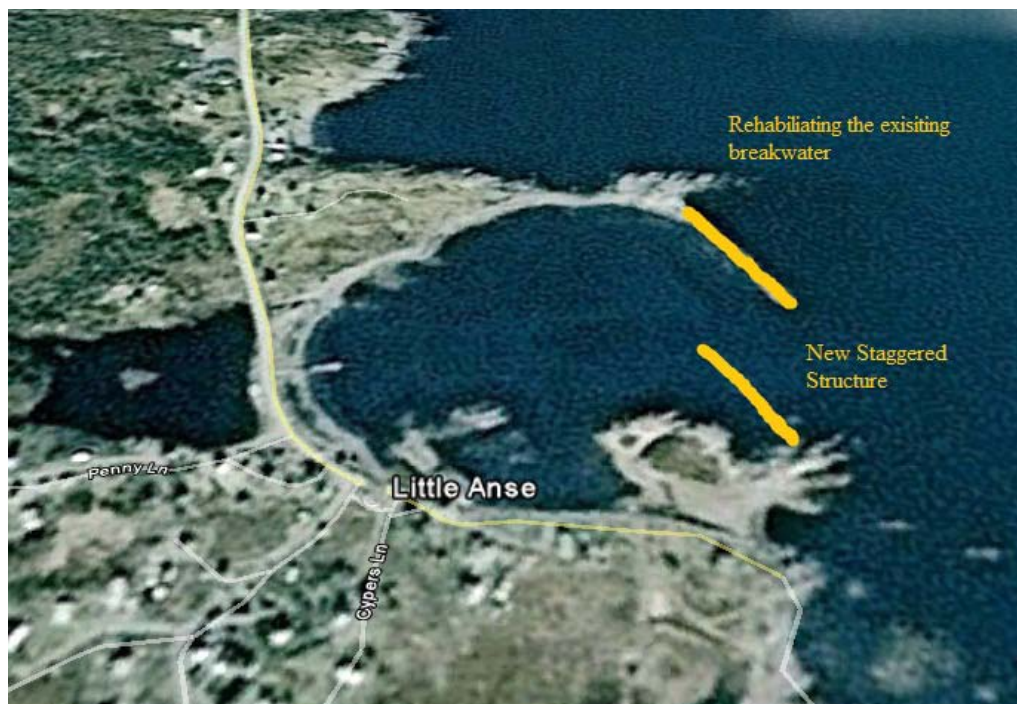
Figure 5.12: A modified opening with a new breakwater arm extending from the south
