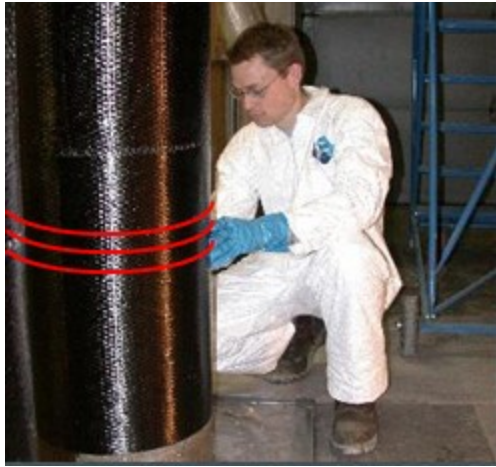
Figure 2-2 Strengthening of existing structures and orientation of fibers
