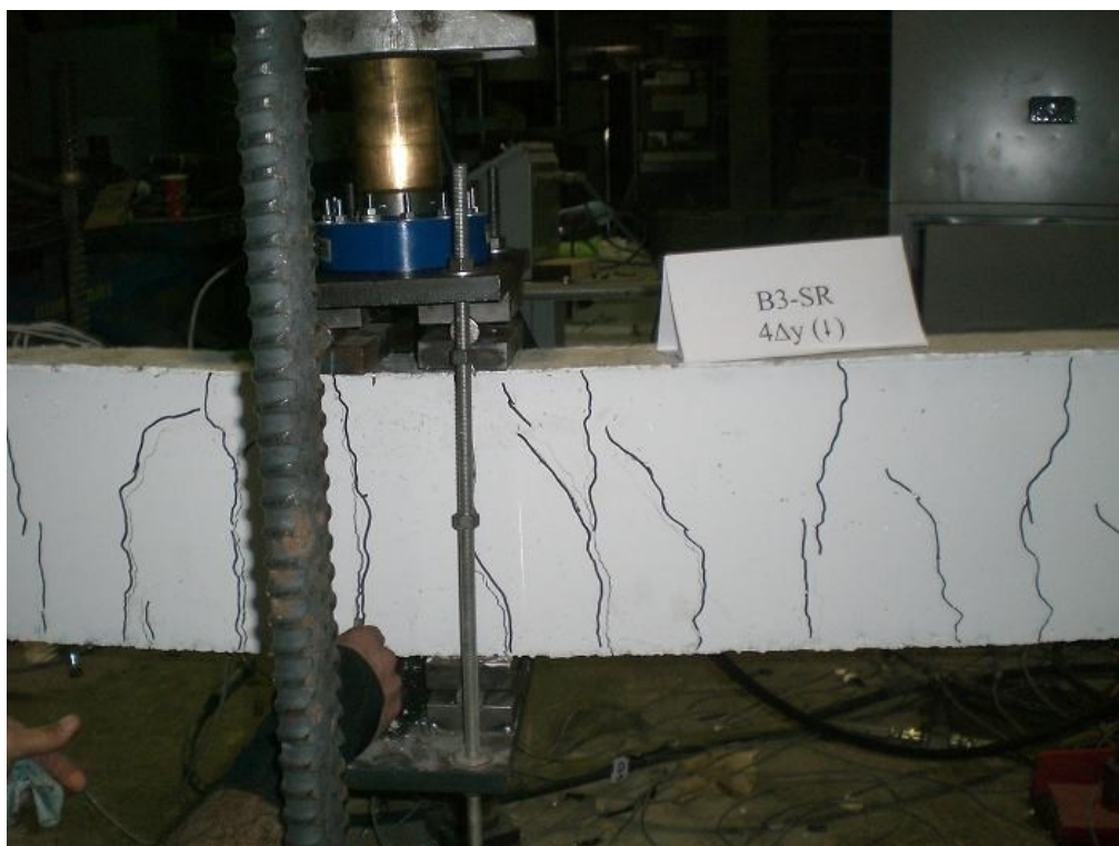
Figure F.14 B3-SR Beam After ( 4\Delta y ) Displacement
