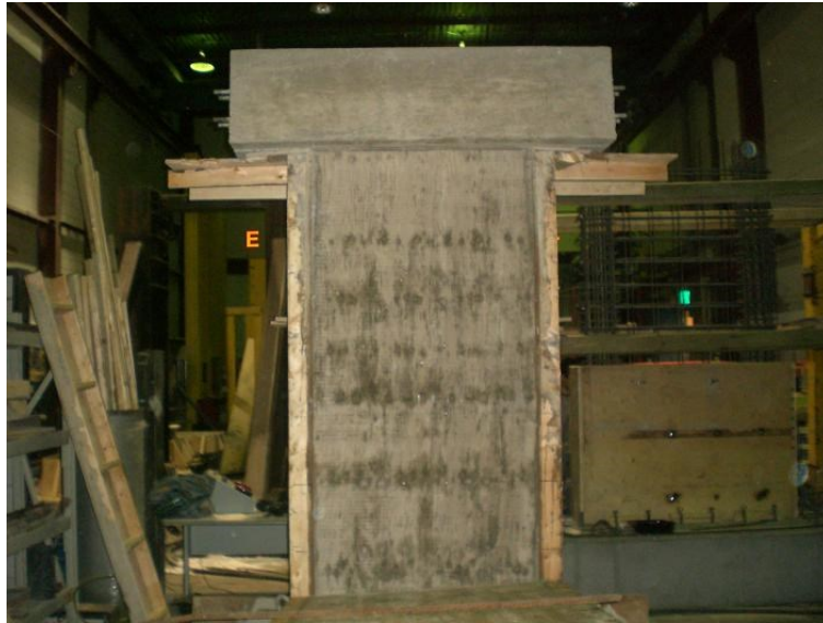
Figure 3.16 Shear Wall Construction (Removal of Formwork)
