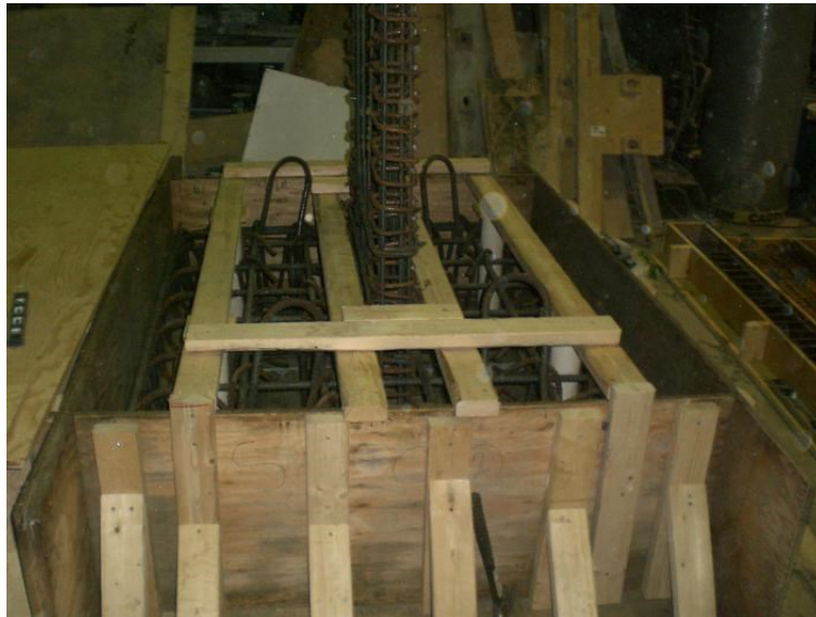
Figure 3.13 Shear Wall Construction (Foundation)
