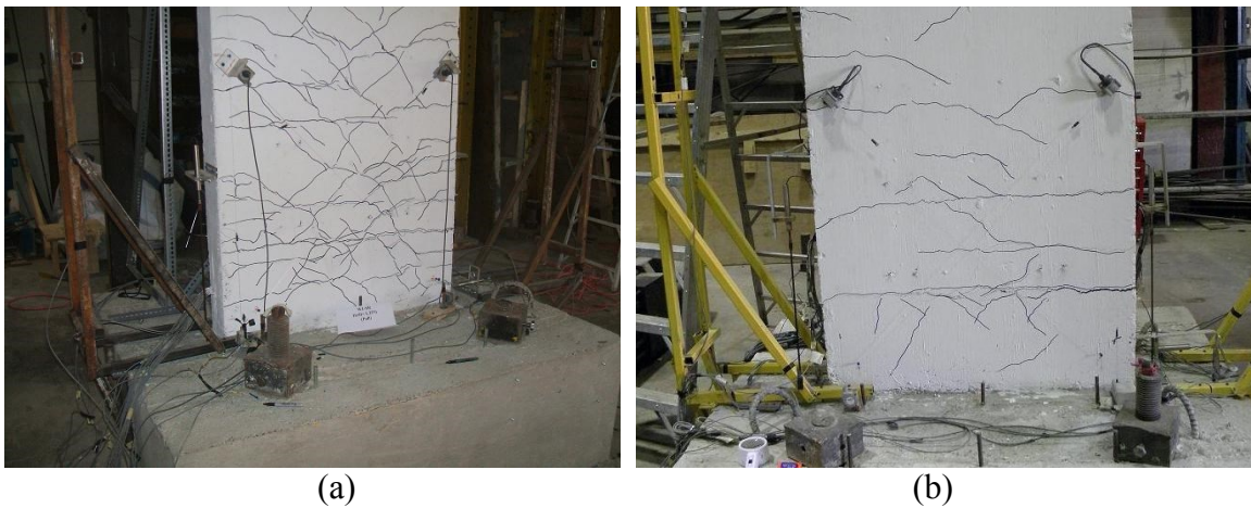
Figure 4.16 Crack Pattern of Test Walls at 1.25% Drift: (a) W1-SR; and (b) W2-NR
