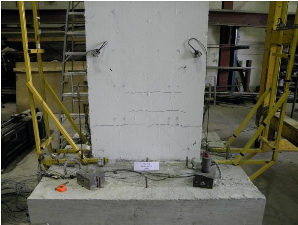
Figure F.45 W2-NR Wall After (0.25%) Drift
