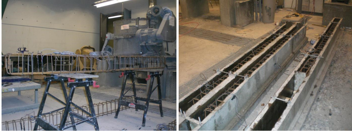
Figure 3.11 Reinforcement Cages and Formwork for Beams
