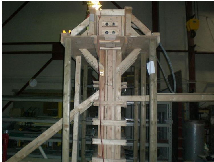
Figure 3.14 Shear Wall Construction (Web Wall and Top Beam)
