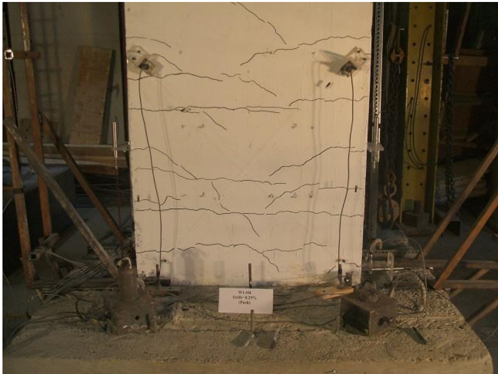
Figure F.37 W1-SR Wall After (0.25%) Drift
