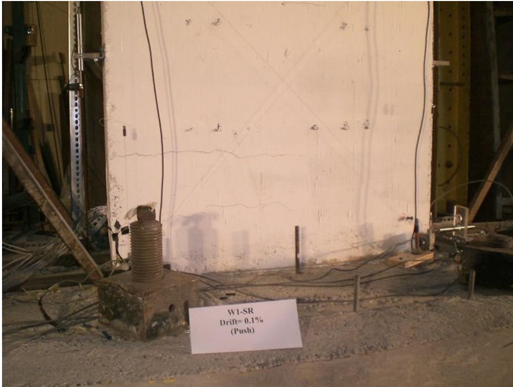
Figure F.35 W1-SR Wall After (0.1%) Drift
