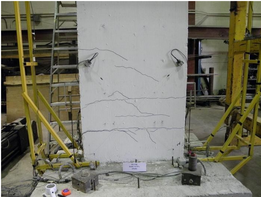
Figure F.47 W2-NR Wall After (0.75%) Drift
