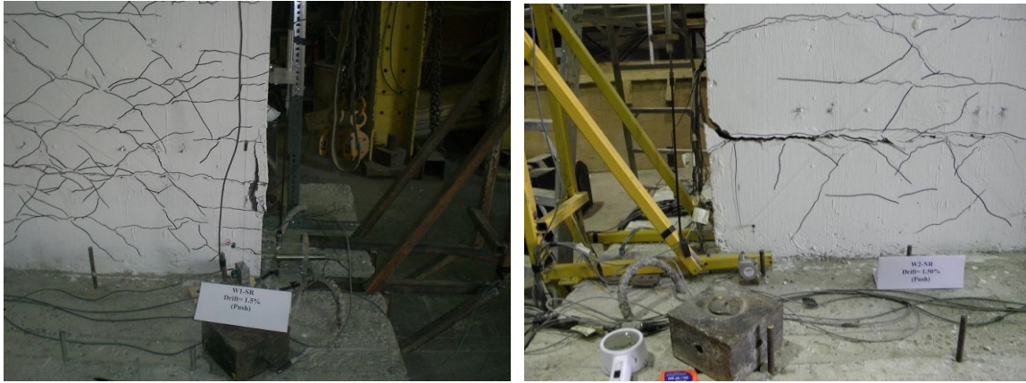
(a) (b) Figure 4.17 Crack Pattern of Test Walls at 1.5% Drift: (a) W1-SR; and (b) W2-NR
