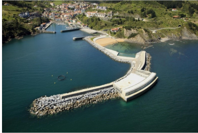
Figure 2.2 – Mutriku Wave Plant [Ente Vasco De La Energia, 2013]
