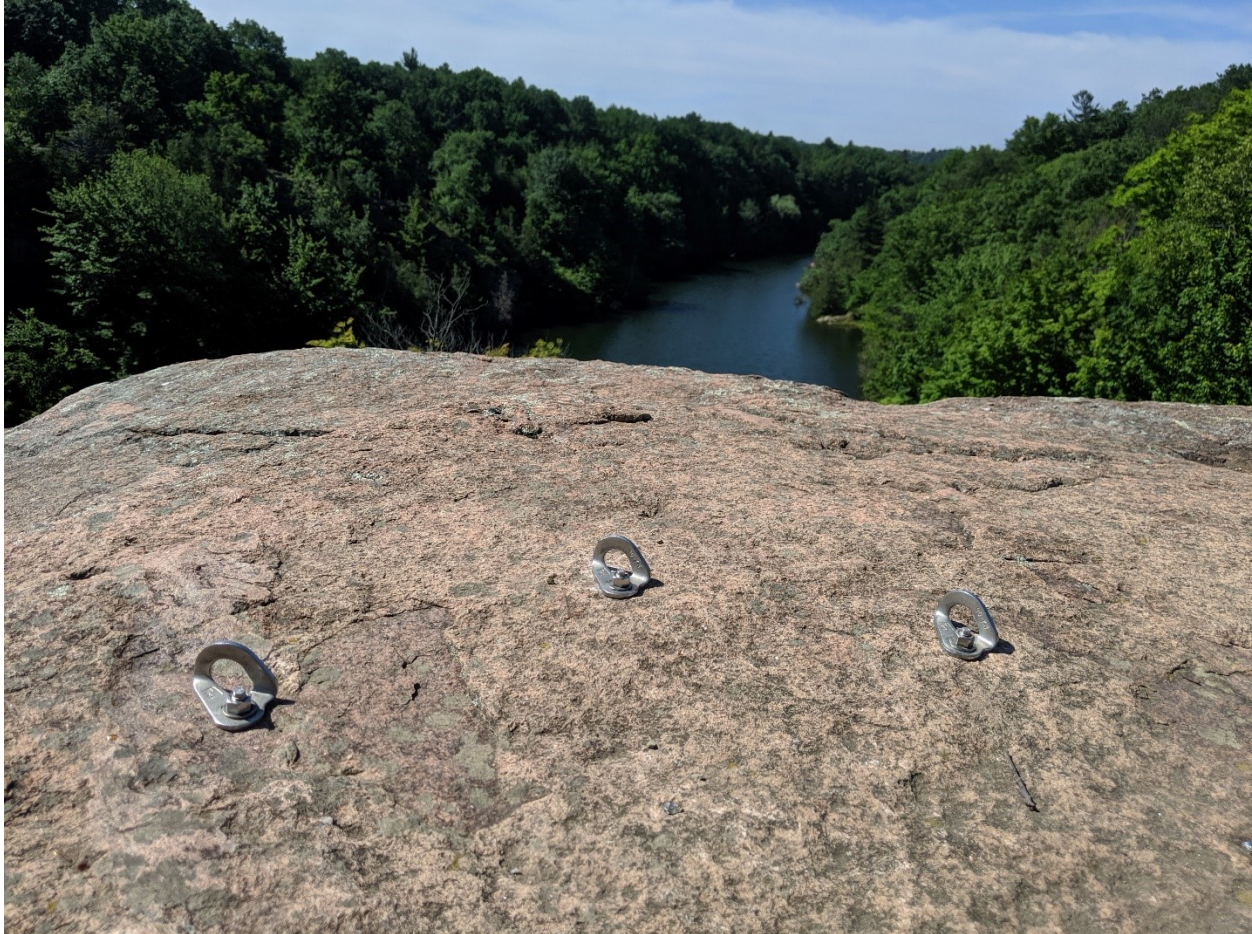
Figure 0.3b. View of the waterway and bolted anchors for top-rope climbing at the Kingston Mills Lock Station (locks 46 to 49) on the Rideau Canal. Photo by the author.
