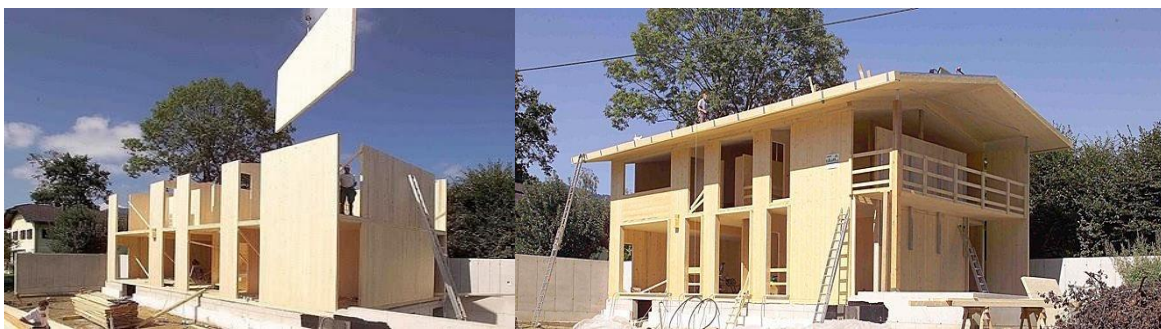
Figure 1-6: Cross Laminated Timber Building (KLH GmbH, 2010)
