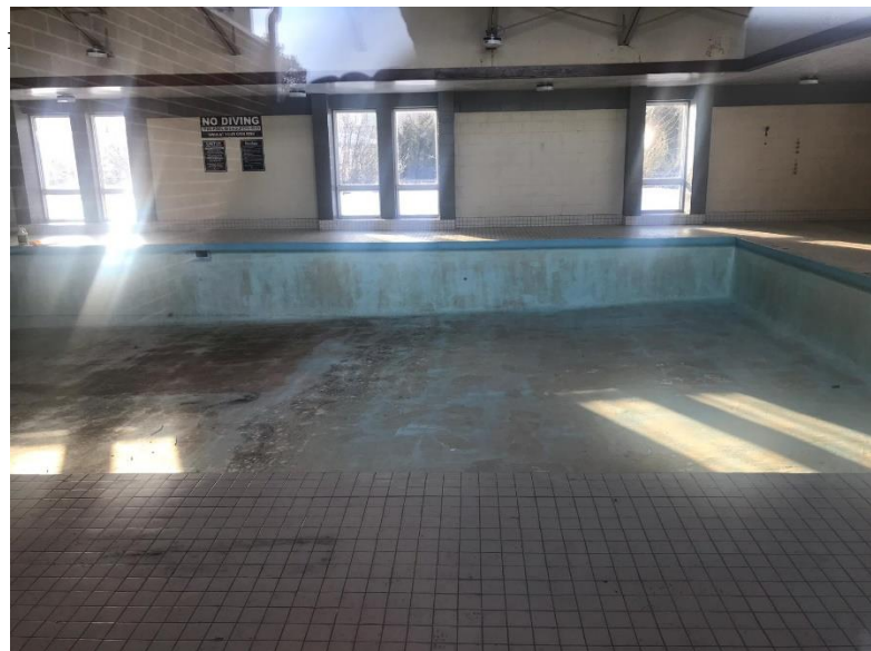
Figure 39: Jarome - Timbercreek Pool
