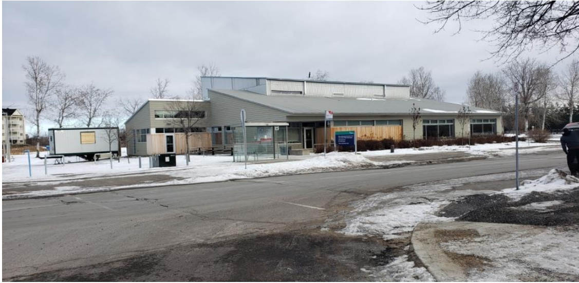
Figure 22: Samira - Albion-Heatherington Community Centre
