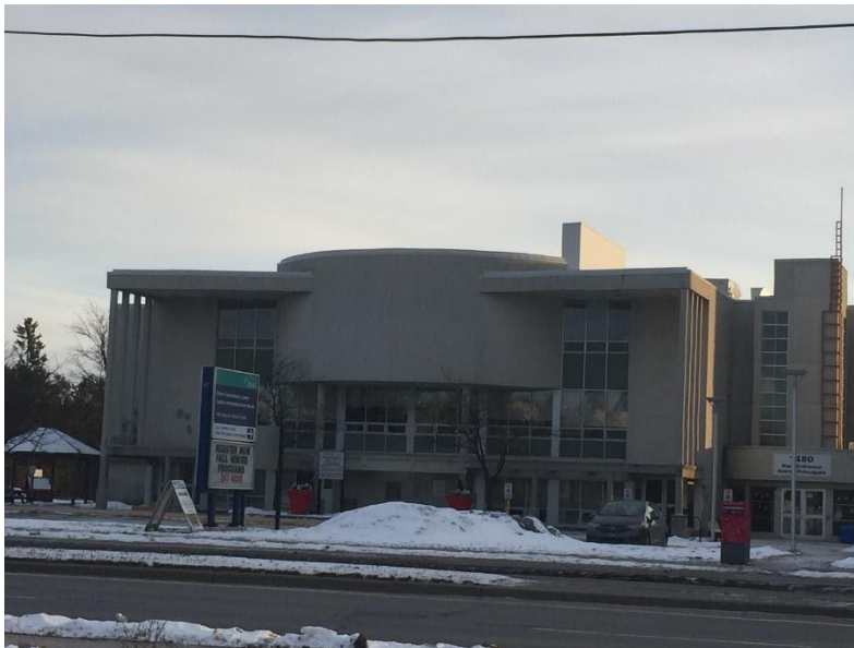
Figure 23: Kinley - Heron Road Community Centre
