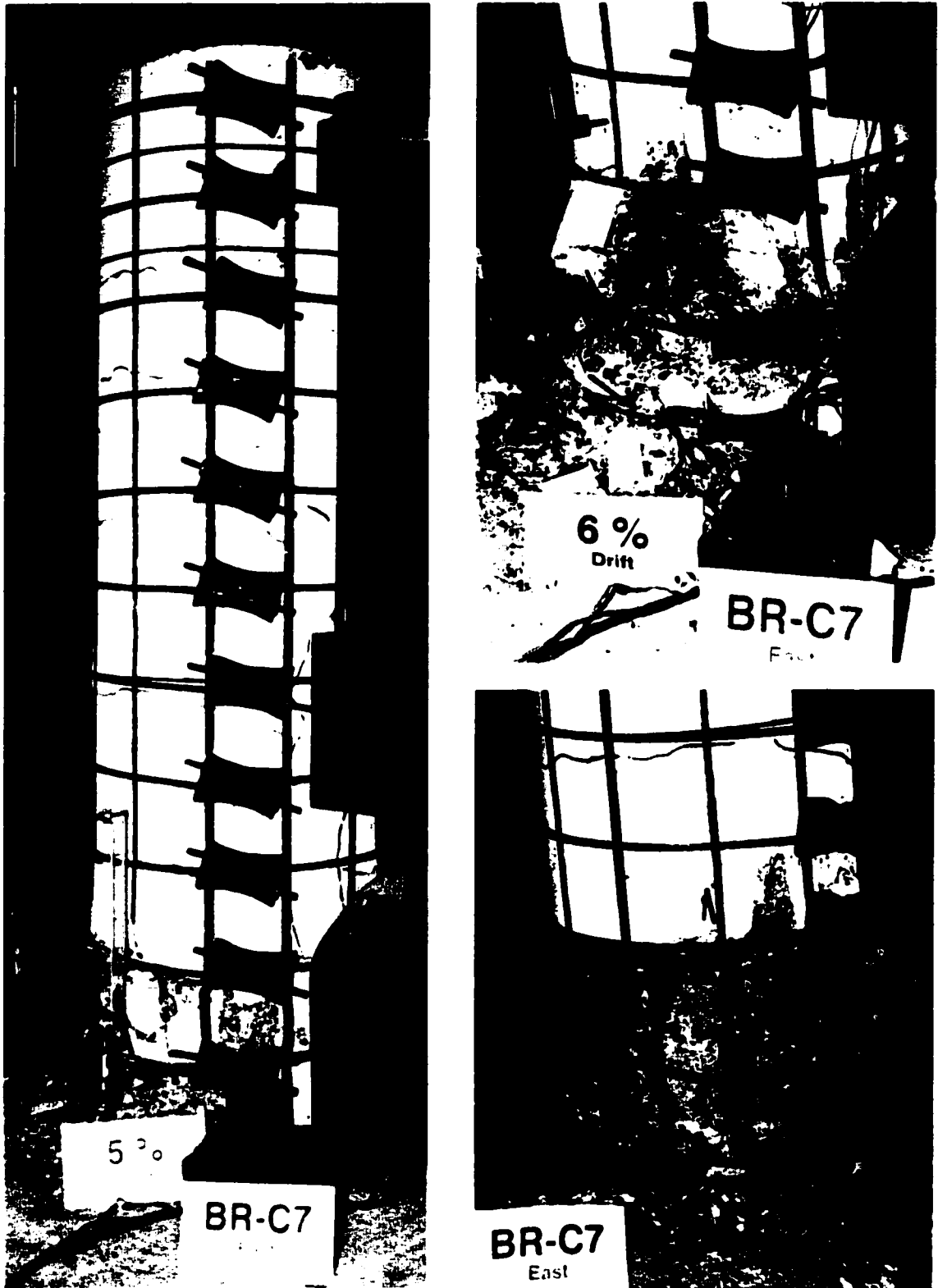
Fig. 3.6c Column BR-C7 at 5% drift (left) and 6% drift (upper right) and at the end of test (lower right)
