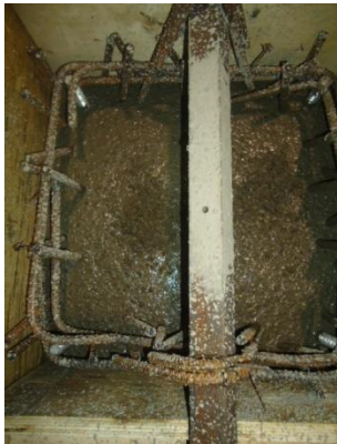
(c) Preparation of concrete footing
