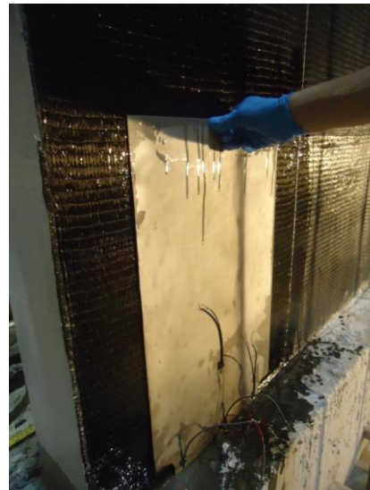
(f) After the placement of anchor
