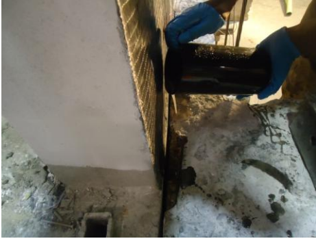
(a) Pouring of epoxy into the concrete slot
