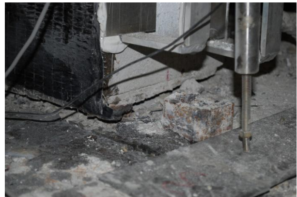
(f) Lifting of wall east end at 0.75% drift
