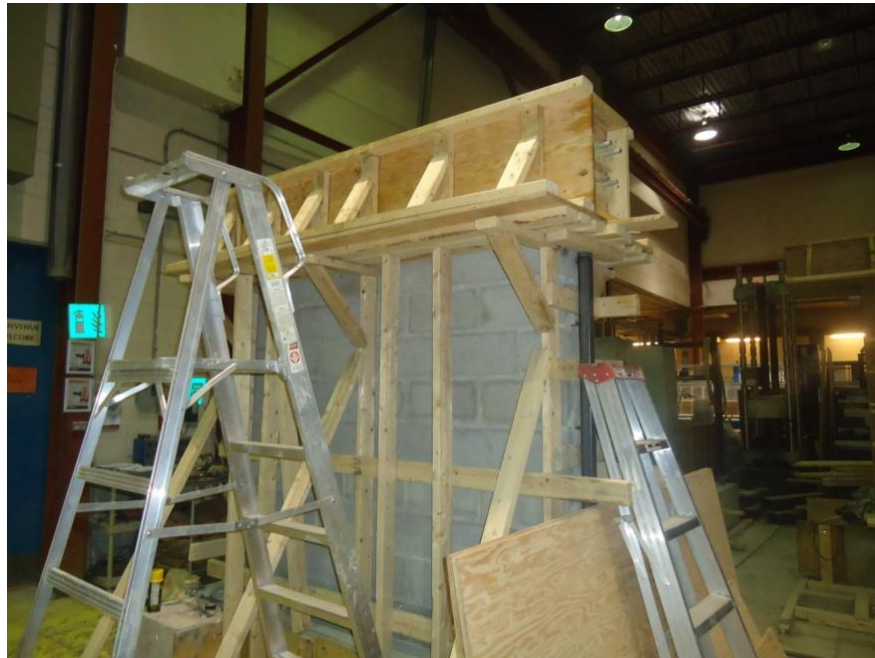
Figure 4.6: Formwork for top beam (PRM Wall)
