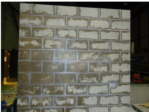
(a) Surface preparation with epoxy putty
