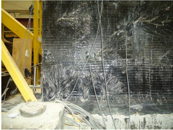
Figure 4.17: FRP anchors after installation on the wall
