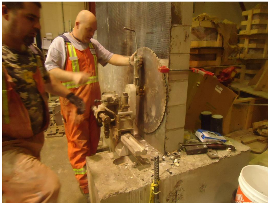
Figure 4.24: Cutting of foundation concrete for anchor placement
