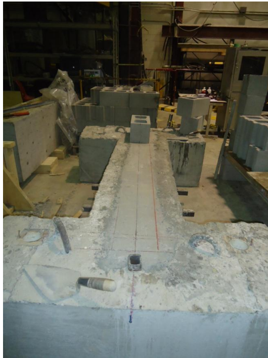
Figure 4.8: Repair of wall foundation
