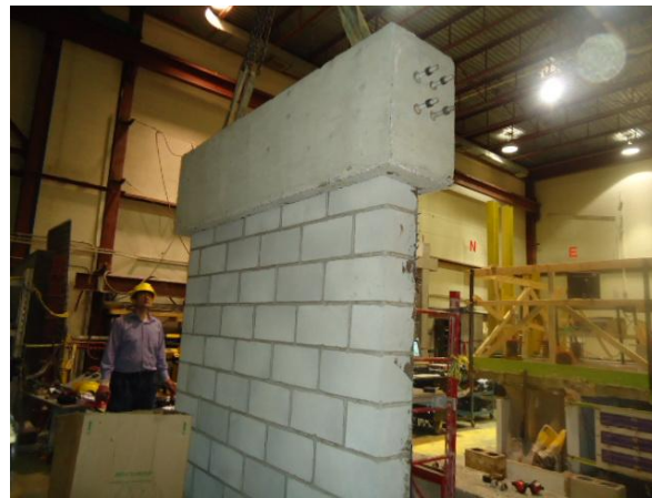
Figure 4.13: URM wall after the placement of top beam
