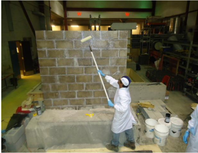
(c) Soaking of wall surface with epoxy
