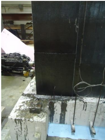
(c) First layer of FRP with vertical fibres
