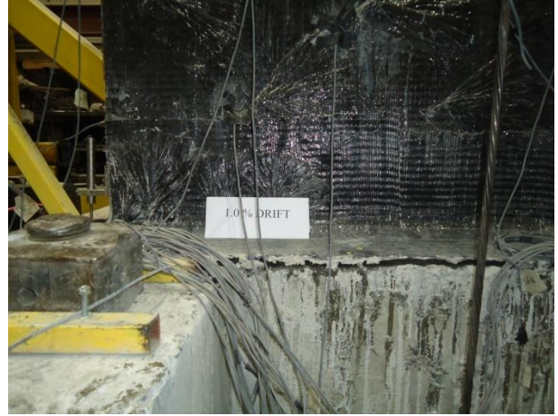
(b) Failure of FRP anchors; 1.0% drift
