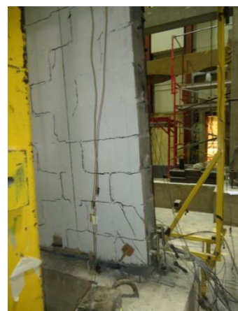
(f) Lifting of west end; 3.5% drift
