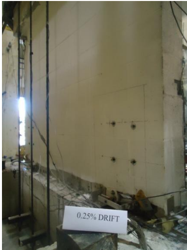
(a) Unretrofitted side of wall at 0.25% drift
