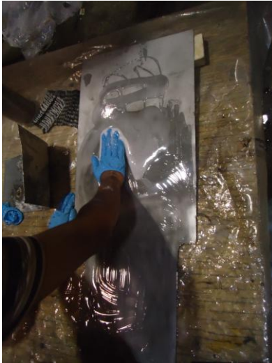
(c) Soaking of the anchor in epoxy
