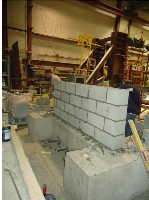
Figure 4.10: URM wall during construction
