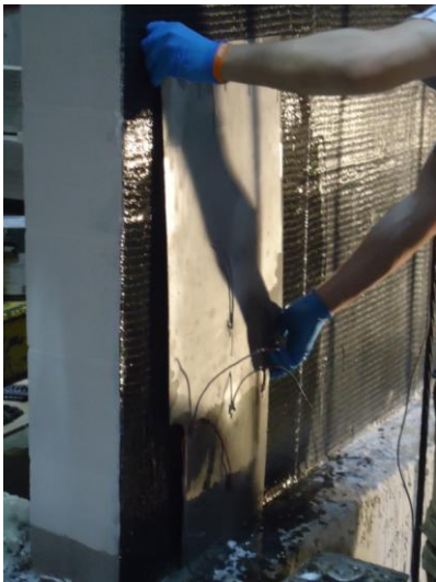
(e) Placement of the anchor in concrete
