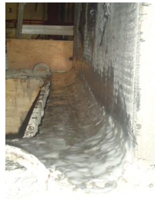
Figure 4.16: Rounded wall footing interface
