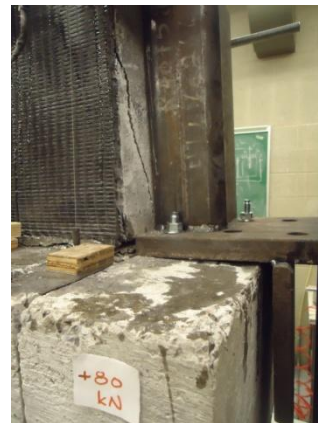
(b) Concrete splitting crack of block
