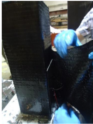
(c) Placement of FRP on anchor
