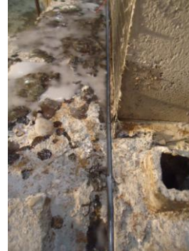
(b) After the placement of epoxy in concrete
