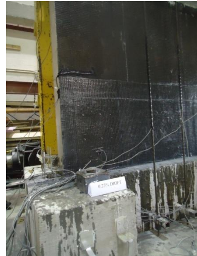
(b) Retrofitted side of wall at 0.25% drift
