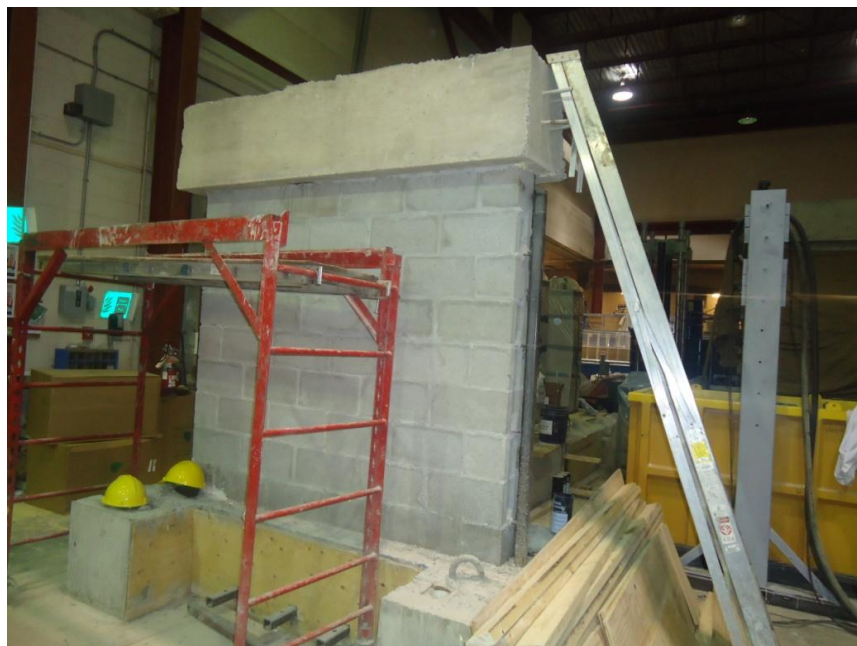
Figure 4.7: PRM Wall after construction
