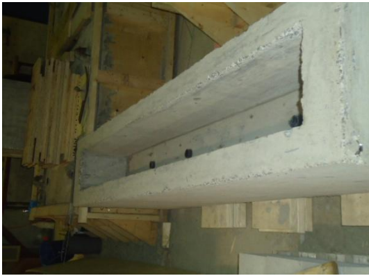
Figure 4.12: The placement of precast top beam on the wall
