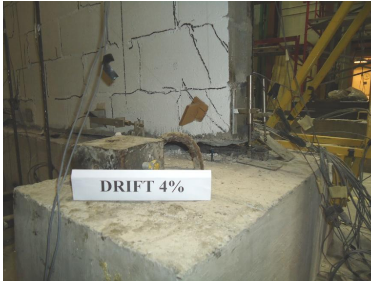
(a) Lifting of west end at 4% drift
