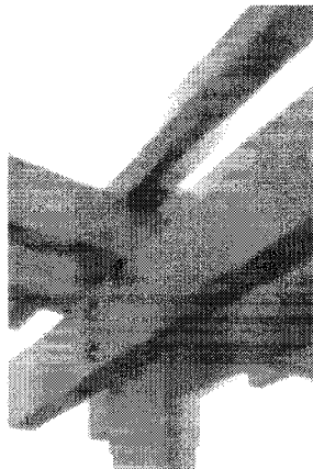
Figure 2.4: Ghosting artifact from using direct blending and feathering of overlapping Ladybug images [48].
