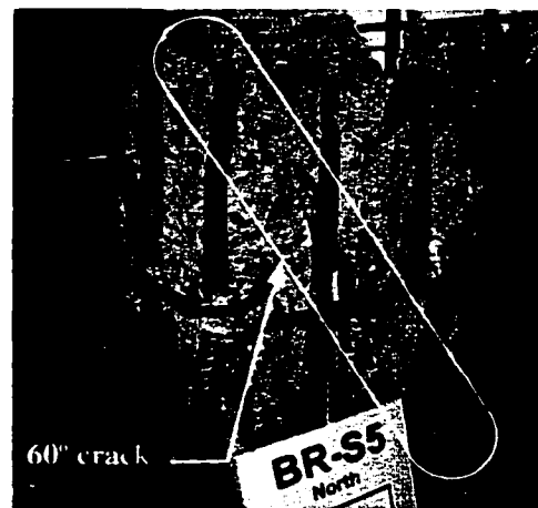
i) After the test (North-East)
