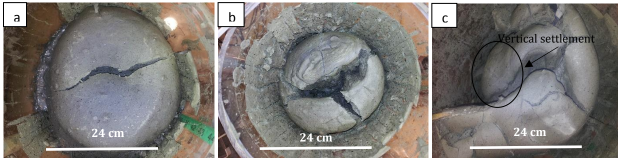
Figure 4.15, Crack formation a) after 10 days b) after 20 days c) after 30 days
