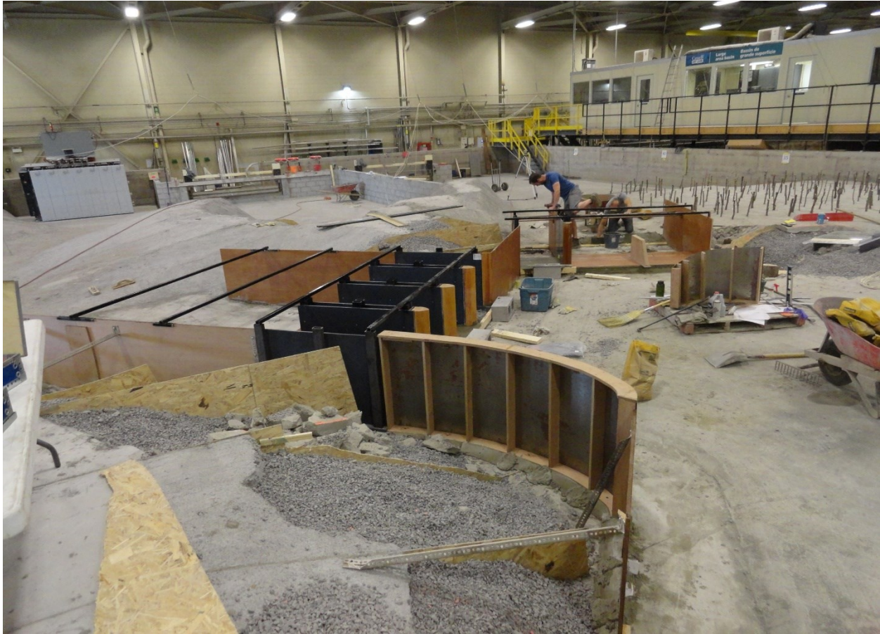
Figure 42: Installation of flow structures and retaining walls (NRC, 2016)
