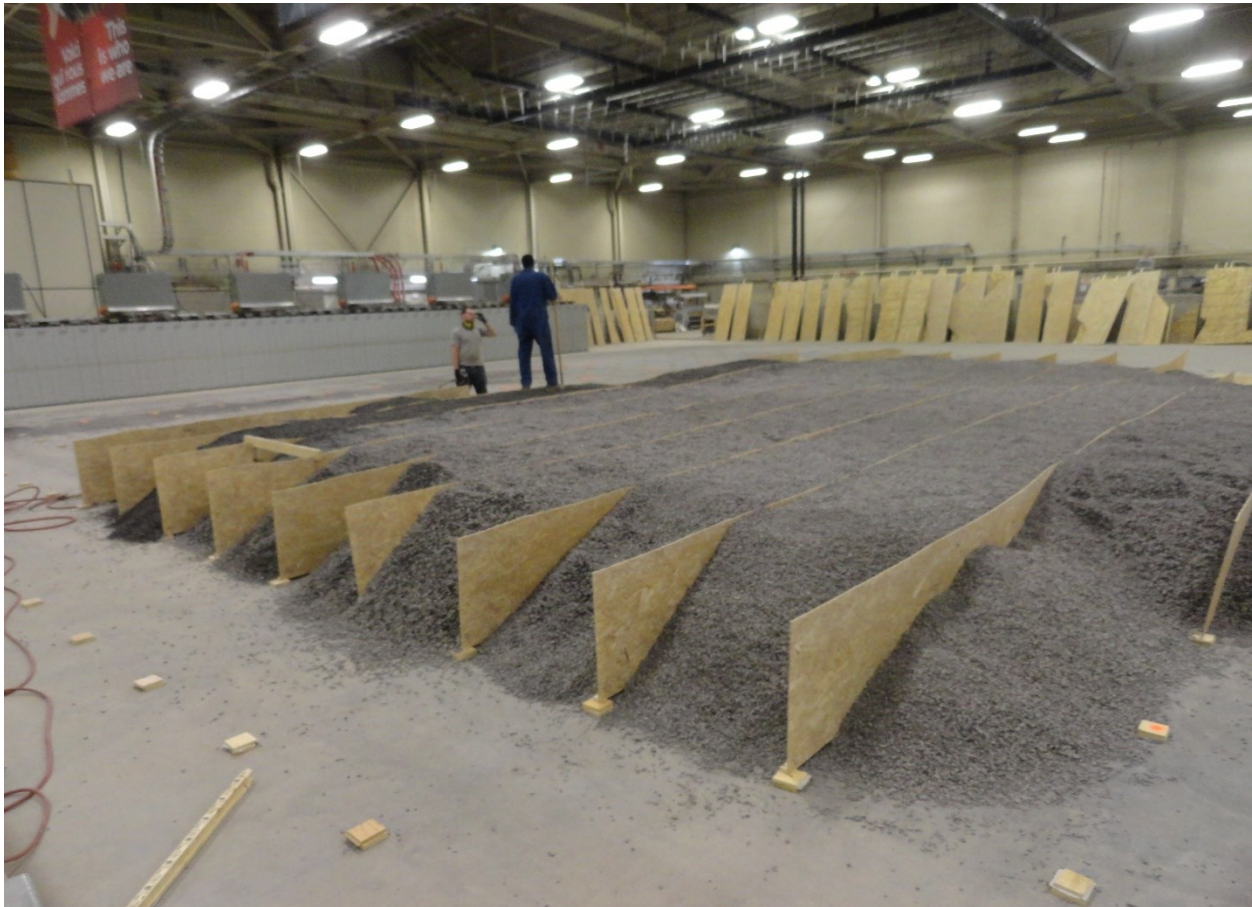
Figure 39: Template installation and backfilling with gravel (NRC, 2016)
