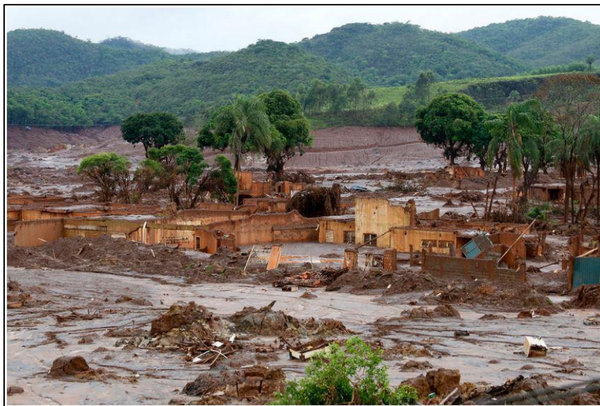
Figure 2.9 The tailing dam failure in Bento Rodrigues Town, Brazil in 2015 (Resourceful Paths 2016)
