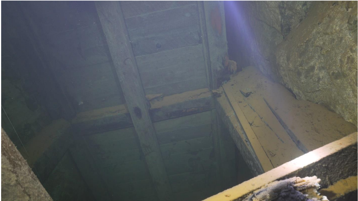
Figure 21 - Elevator shaft (Photo by Kevin Brown)
