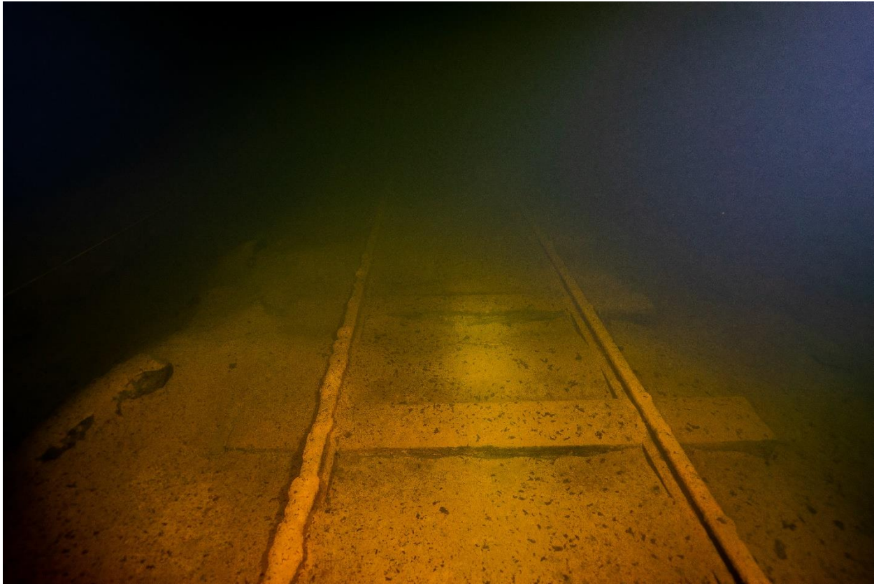
Figure 25 - Train track leading to the exit in Forsyth Mine (Photo by Kevin Brown)
