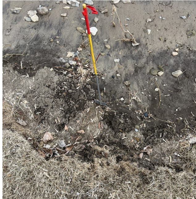
Fig. 2 Erosion rod installed at Mariatown Bay shoreline (June 2022).
