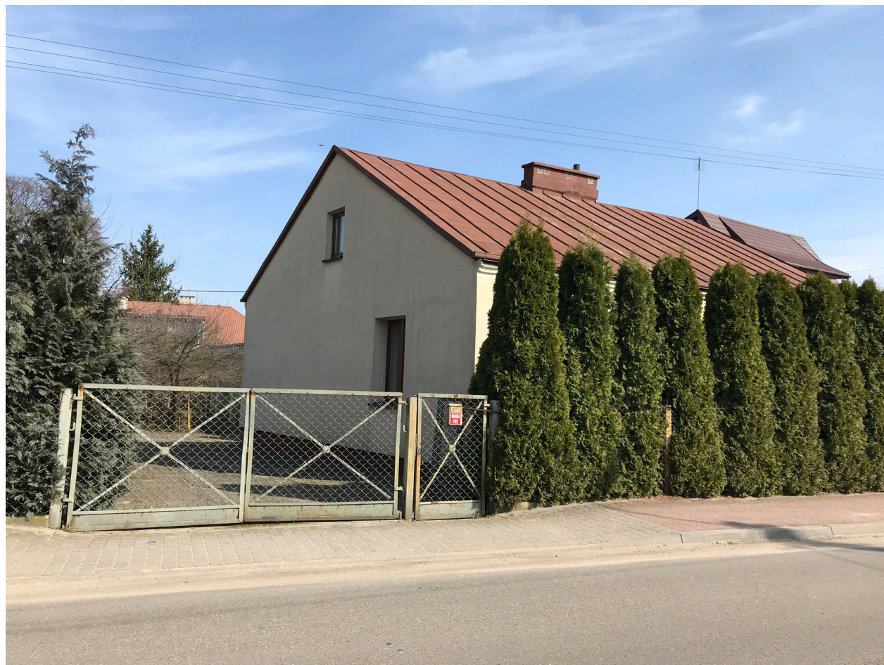
Image 3. The house in which Aaron Elster and his sister Irena hid with the Górskis. While the structure stands in its original form, the roof was reconstructed after it was destroyed by Russian bombings in 1944. Source: Photo by author, March 30, 2019.
