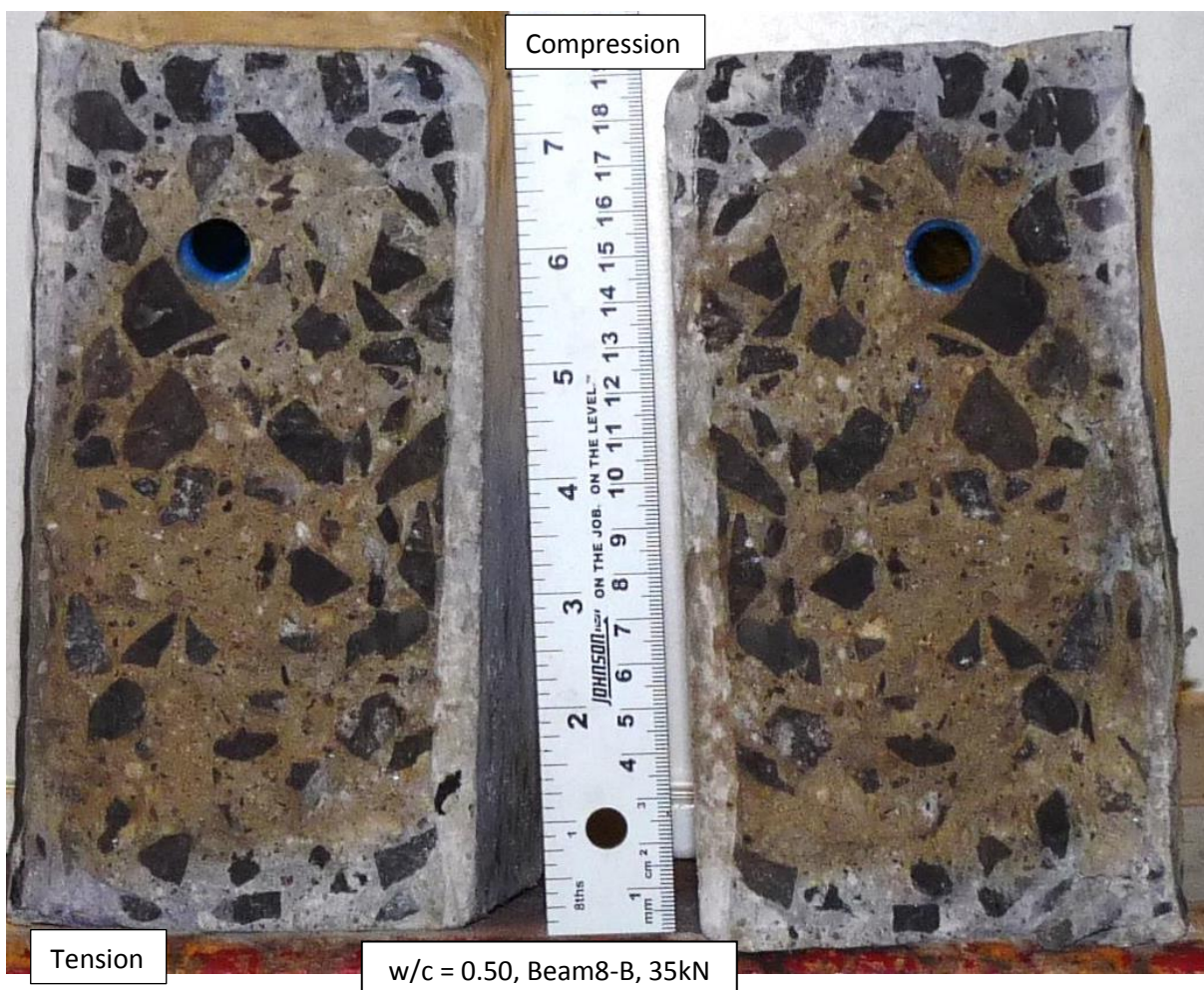
Figure C.30: Chloride penetration depths for beam 8; section B8-B ( w/c = 0.50 , 35 kN)
