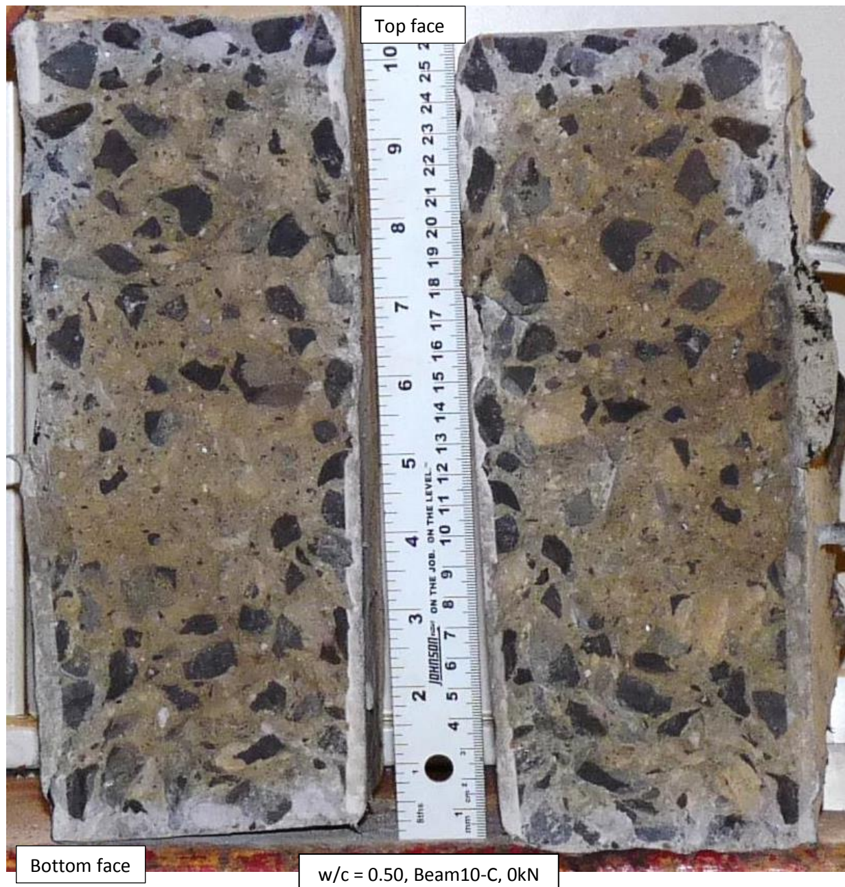
Figure C.39: Chloride penetration depths for beam 10; section B10-B ( w/c = 0.50 , 0 kN)
