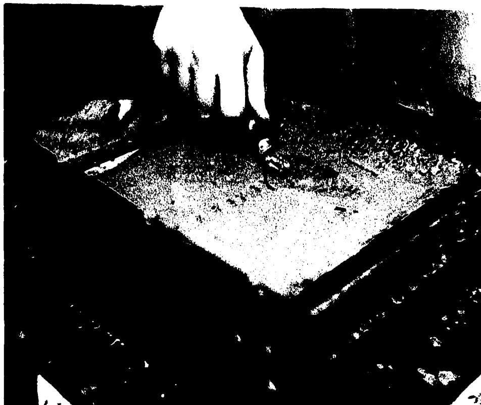
PLATE 3.5 - TROWEL FINISH OF CONCRETE SLABS
