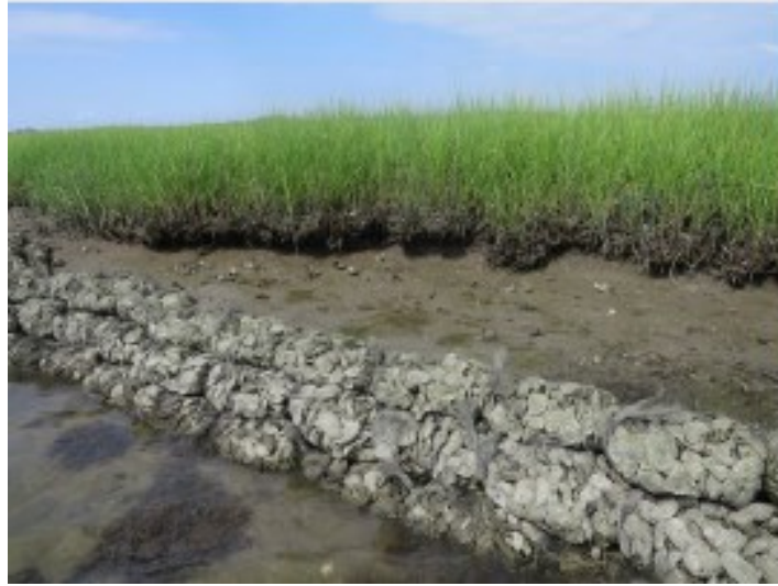
Figure 2-1. Bagged shells as an oyster reef in Virginia (Morris et al., 2019)
