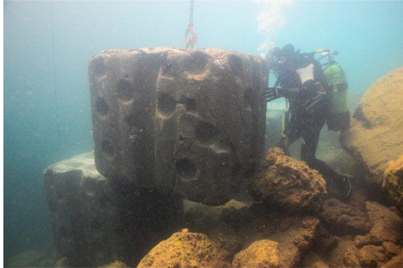
Figure 2-10. EConcrete Antifers during construction in Polinom Port, Haifa (Ido et al., 2015)
