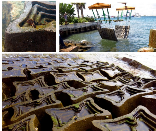
Figure 2-12. Ecological Articulated Concrete Marine Mattress (EConcrete, 2021)
