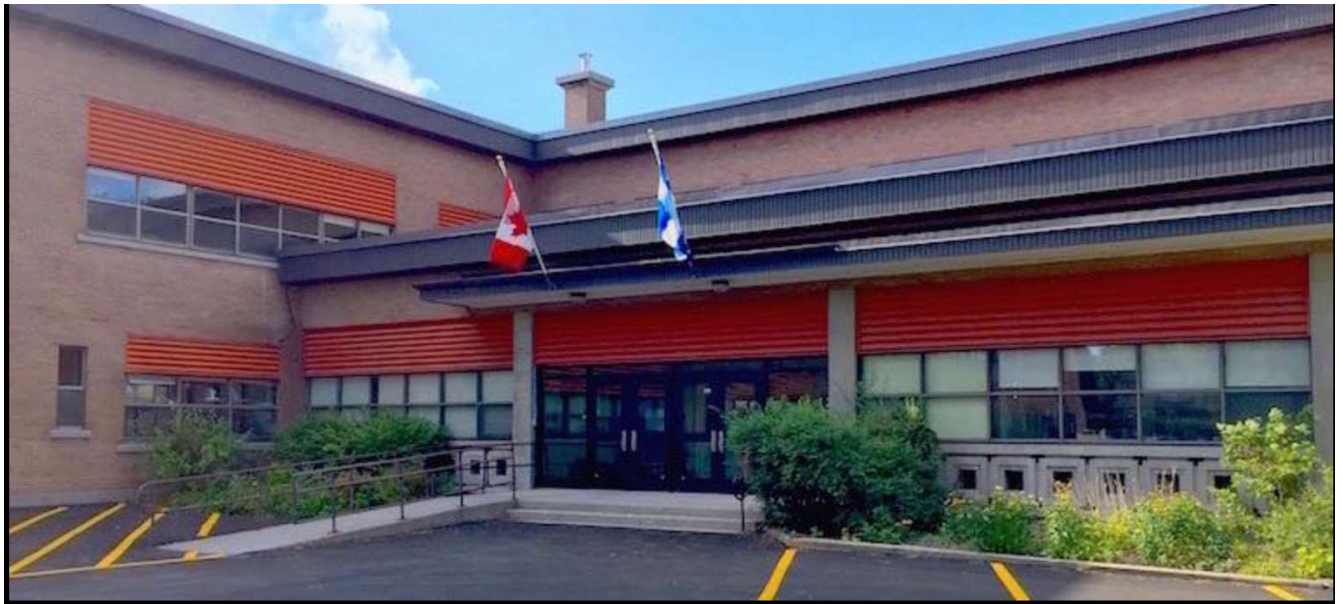
Figure 24: Pierre Elliot Trudeau Elementary School (Source: own photo).
