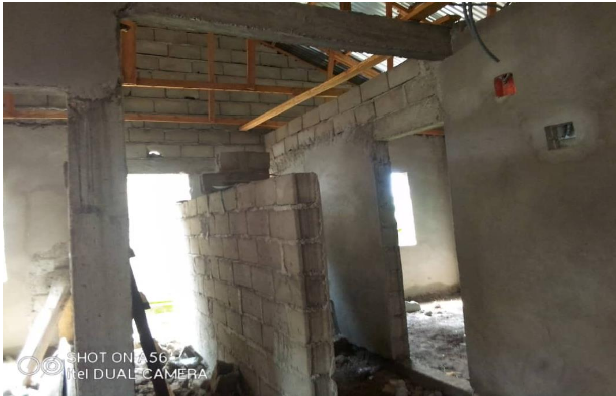
Figure 9.1. Uncompleted maternity building extension from PBF bonus, Tiko
