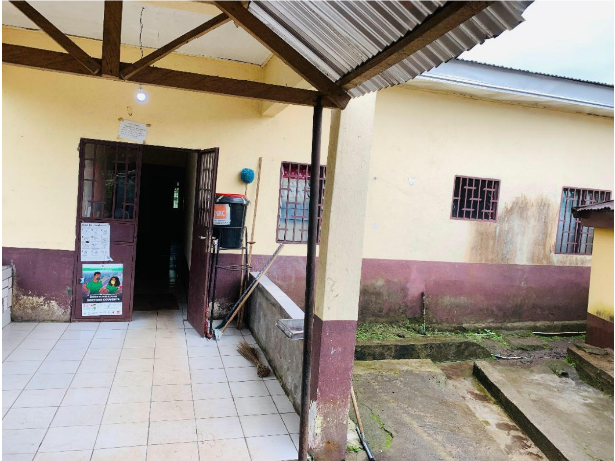
Figure 8.1. Maternity extension partially built with PBF bonus at public health facility, Buea
