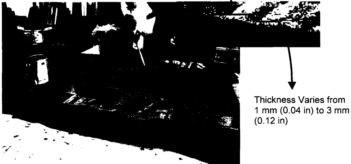
Figure 9.5 Variation in the Application of the Adhesive Thickness
