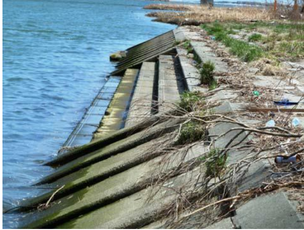
Figure 51: Concrete Sloped Banks of the Natori River (Robertson, ASCE 2010)
