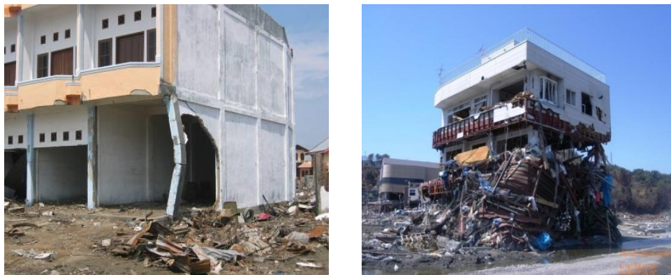
Figure 1: Structures damaged by tsunami impact forces and debris (Left: Saatcioglu and Nistor (2006), Right: Nistor (2011))
