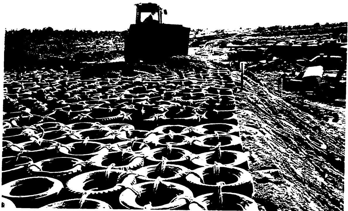
Figure 5.16. Infilling of the tire mat reinforcements.
