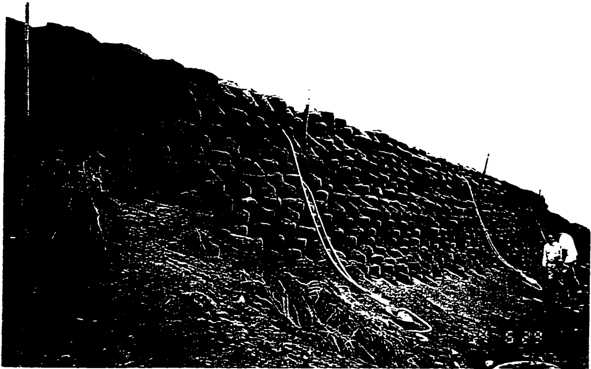
Figure 5.19. Completion of the tire retaining wall (height 4m).
