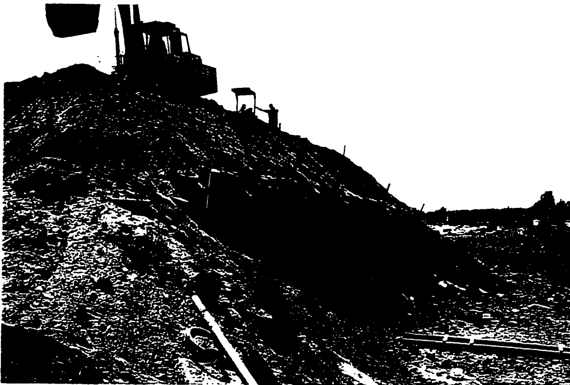
Figure 5.22. The placement of the surcharge load.
