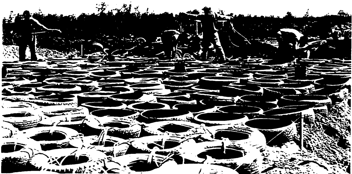
Figure 5.15. A series of photographs showing the fabrication of the tire mats.
