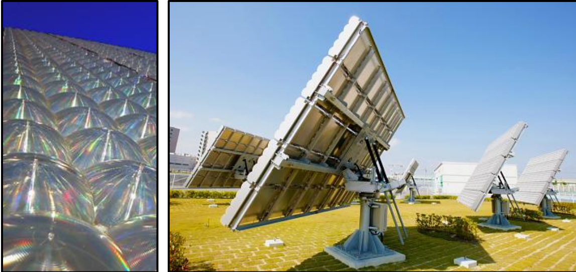
Figure 1-23: Daido Steel dome shaped Fresnel Lenses designed to minimize chromatic aberration and maintain a short focal length. Pilot plant deployed in Tokoname-city, Aichi Prefecture, Japan has been in operation since February 2009 [39].
