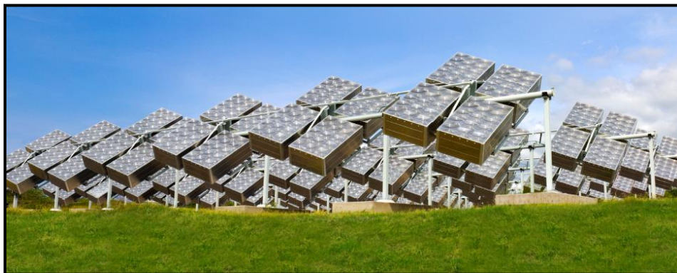
Figure 1-22: Emcore terrestrial CPV deployment with tilt and roll tracking system and silicone-on-glass lens concentrating at 1090x the intensity of the sun [37].
