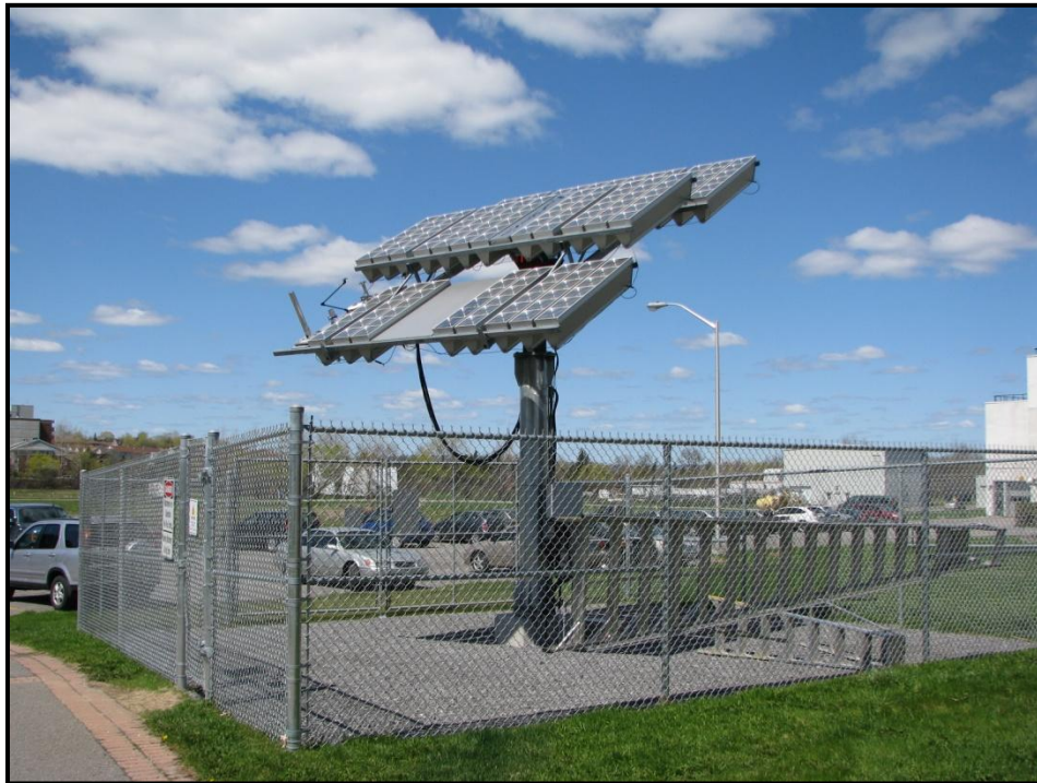
Figure 1-16: The SUNRISE demonstrator May 9 th , 2011. The SUNRISE demonstrator holds high-efficiency quantum-dot-enhanced triple-junction solar cells designed and manufactured by Cyrium Technologies Inc. that have been integrated into OPEL Solar MK-I Fresnel-lens-based 550x concentrating modules that are pointed at the sun with an OPEL Solar dual axis tracker that is manufactured by Trackers FEiNA.
