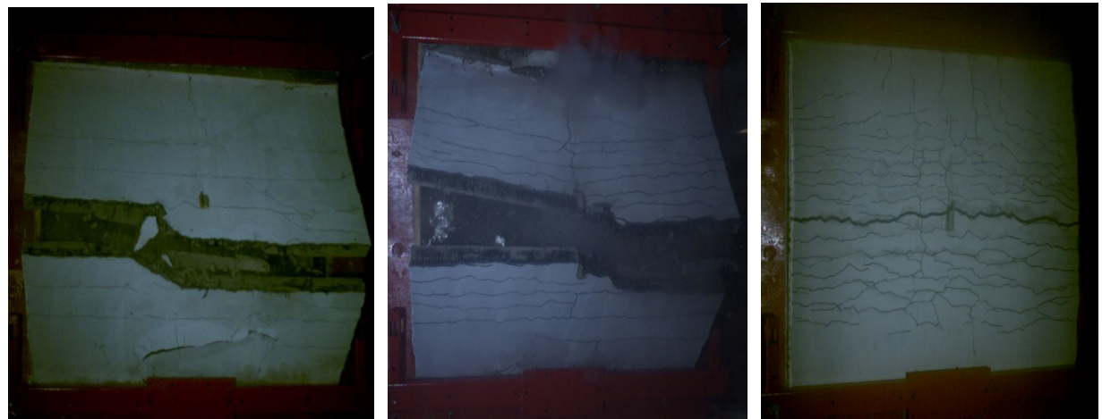
Figure 5-11. Retrofit Ratio Damage Comparison: RCL-NC-1, RCL-YC-2, RCL-YC-3 (continuation)
