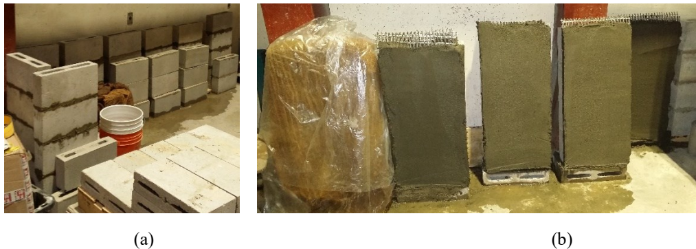
Figure 3-24. Specimen preparation: (a) Construction, (b) Installation of FRCM composite
