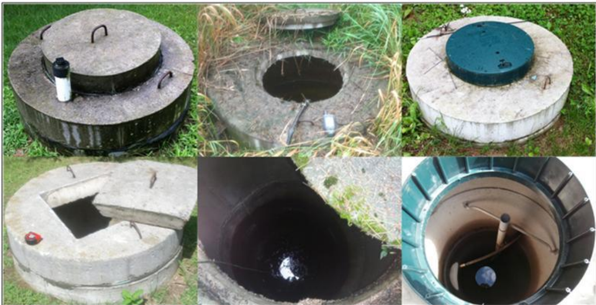
Figure 4-2. Dug wells encountered with concrete caps (left) and vermin-proof caps (right).
