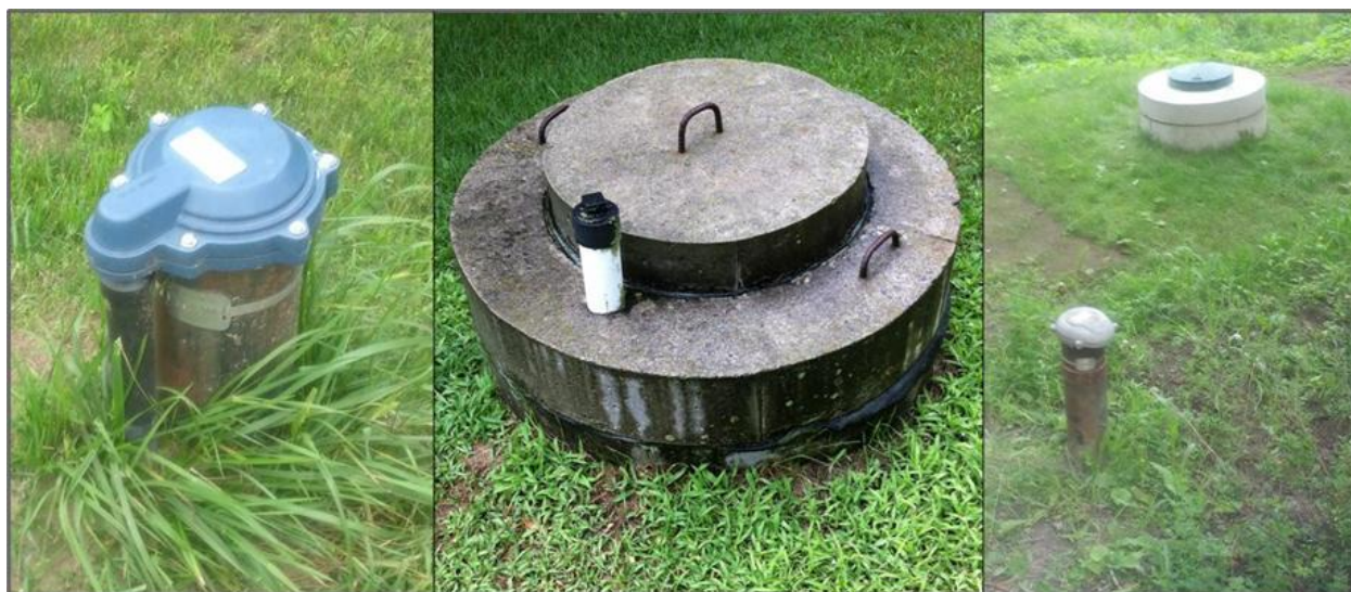
Figure 3-1. Photos of a drilled well (left) and a dug well (middle) with a side by side comparison for scale (right).
