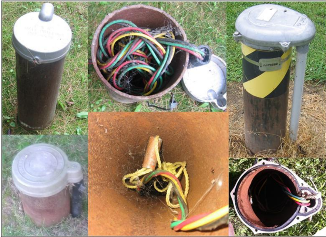
Figure 4-1. Drilled Wells encountered with standard steel caps (left and middle) and vermin-proof caps (right).
