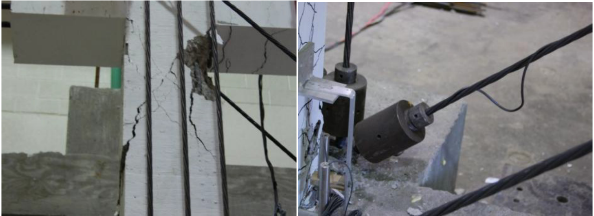
Fig. 4.16 Damage during the last cycle of 2.5% drift; (a) diagonal tension failure of column at the top, (b) ruptured wire of a strand
