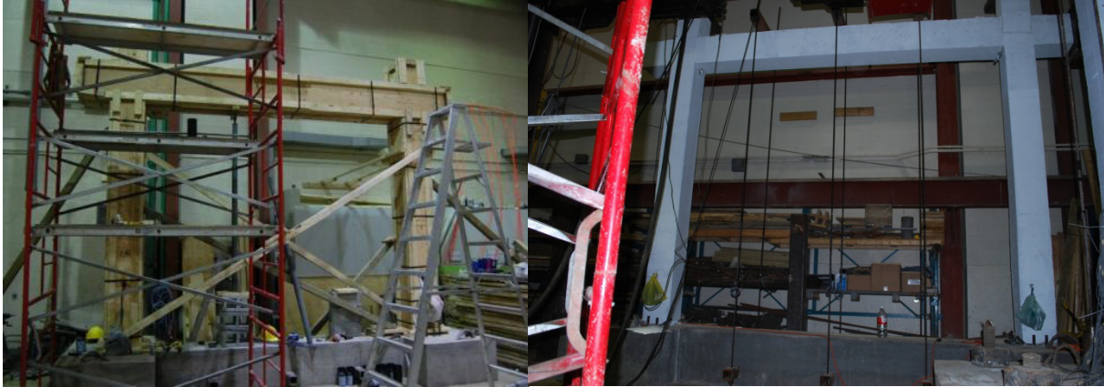
Fig. 3.6 Frame formwork and frame after formwork removal
