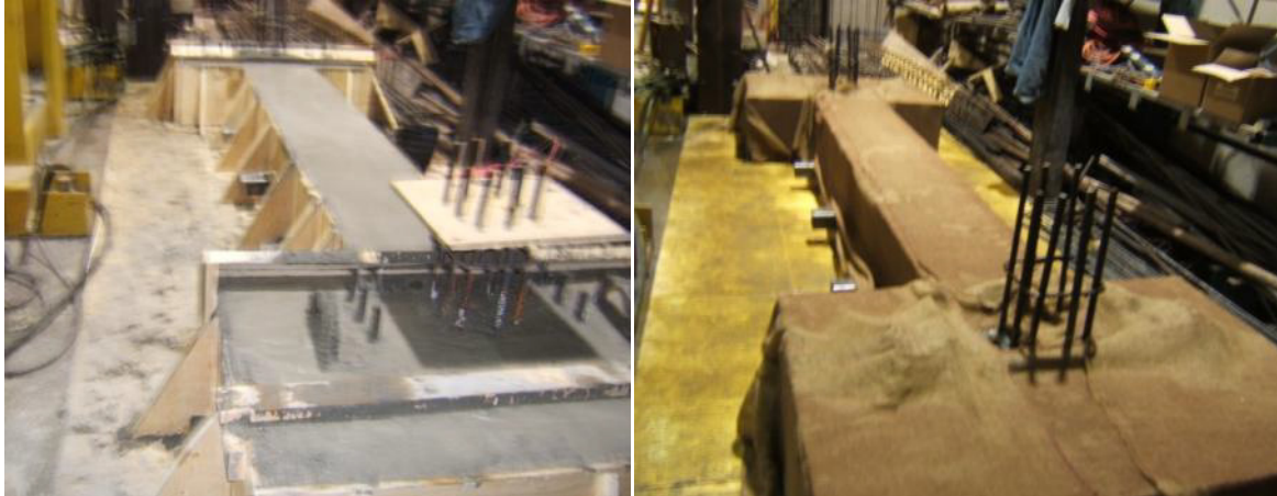
a) Fresh concrete after finishing
