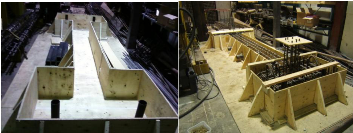
(a) Formwork with 3 inch pipes
