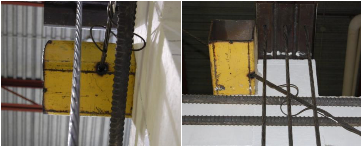
Fig. 4. 9 Ruptured diagonal prestressing tendon during testing of Frame No. 2
