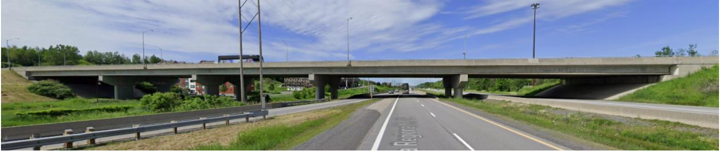
Figure B.3 Side View of Overpass Showing Five Spans (Google Maps)
