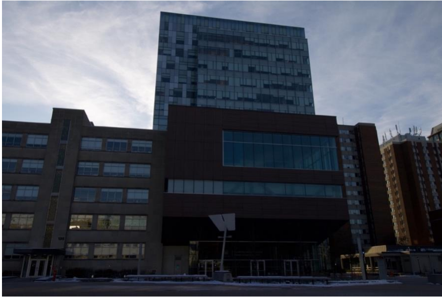
Figure C.1 FSS Building from the Front
