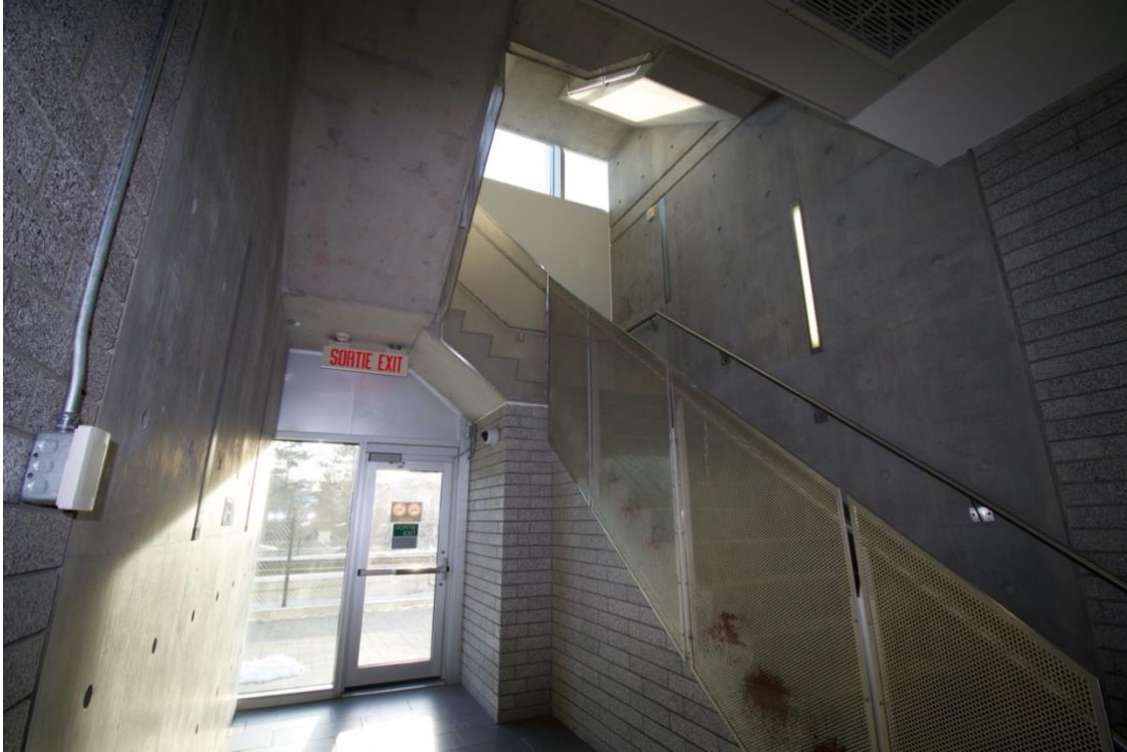
Figure C.6 FSS Building from Inside (Staircase)
