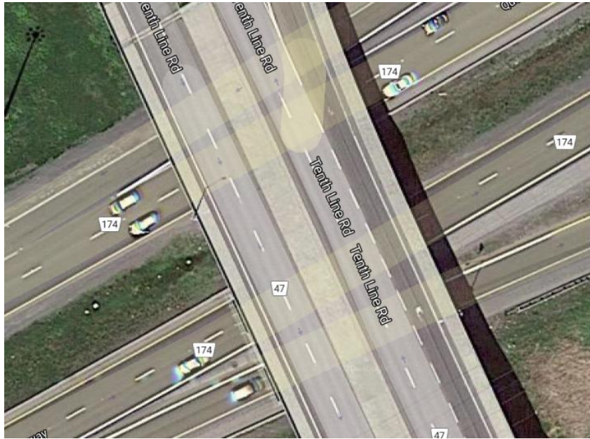
Figure B.1 Tenth Line Road Overpass – Satellite View (Google Maps)
