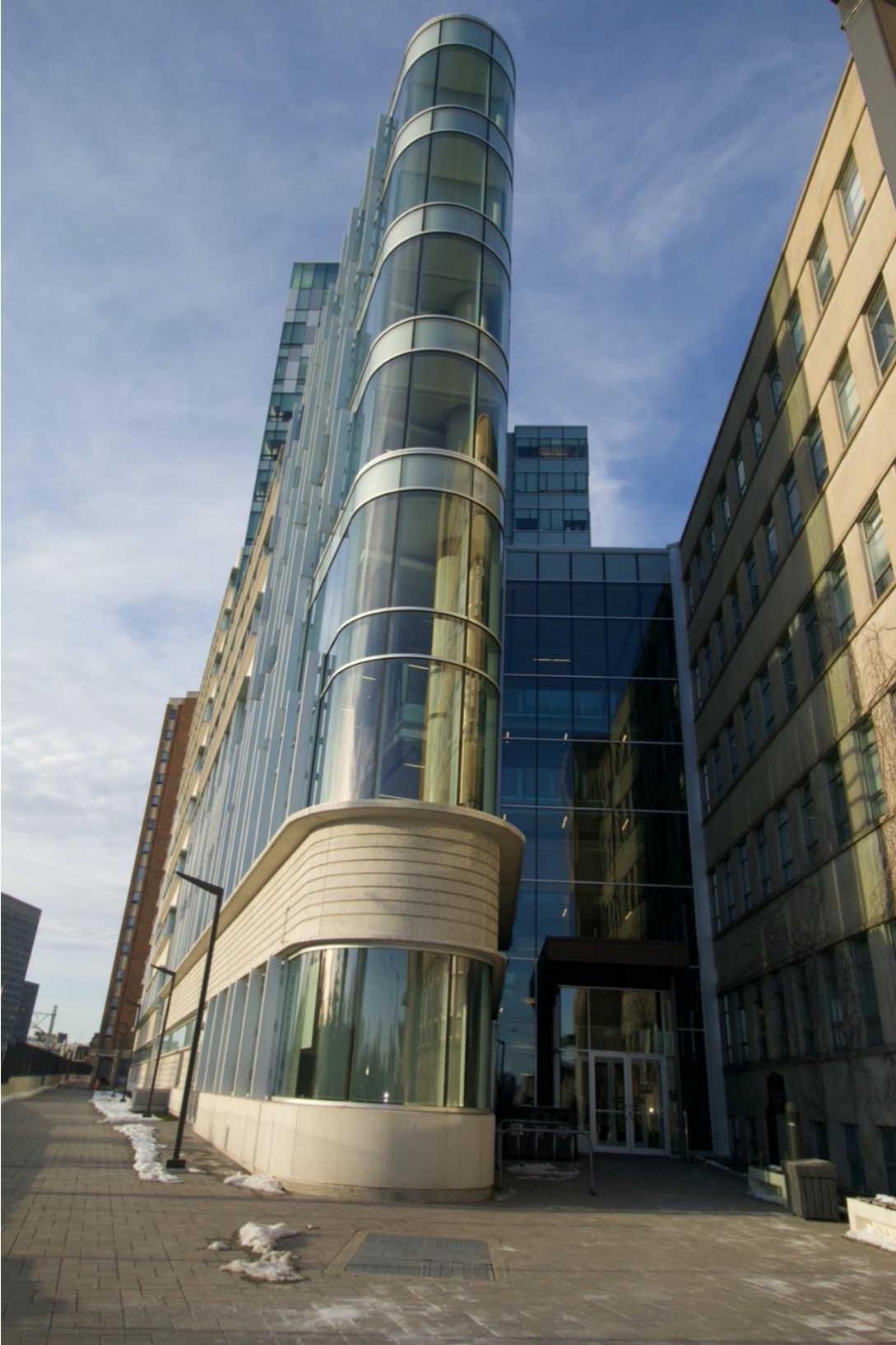
Figure C.3 FSS Building from Back (Connection to Vanier Hall)
