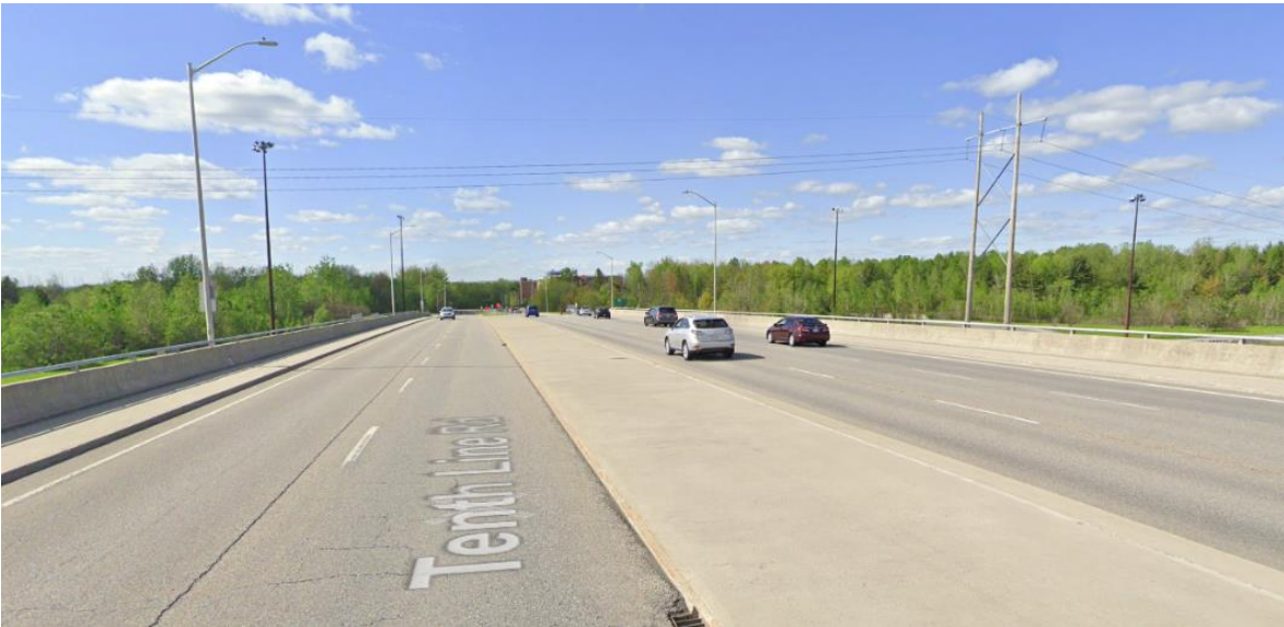
Figure B.2 View on Overpass Showing Five Lanes (Google Maps)
