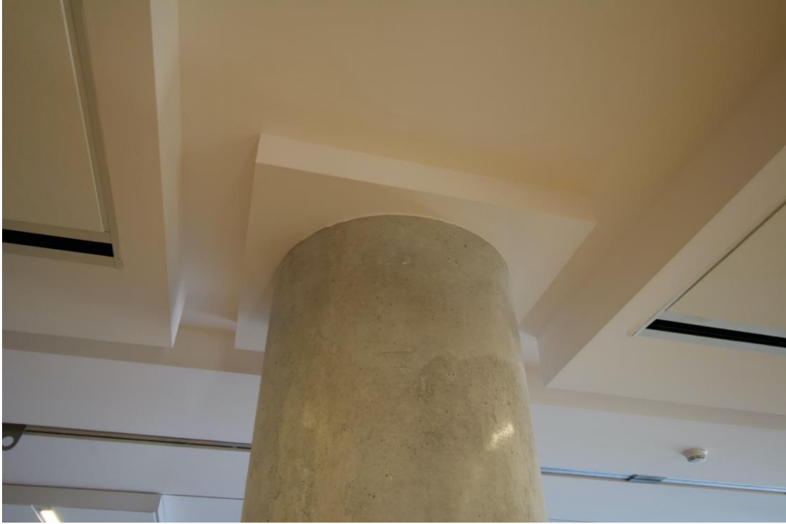
Figure C.10 FSS Building from Inside
