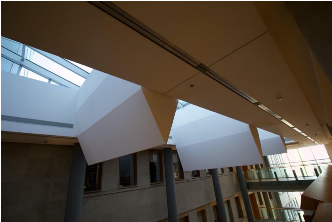
Figure C.9 FSS Building from Inside
