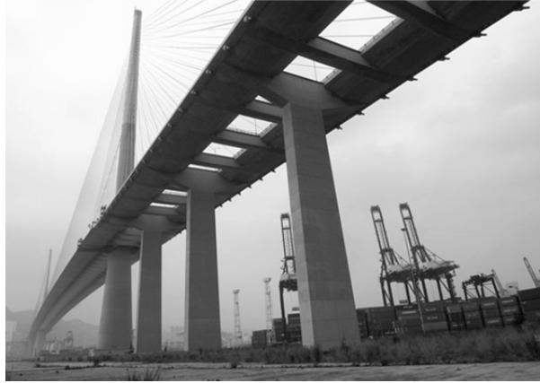
Figure 3.10: Concrete back-span and piers of Stonecutters Cable-stayed Bridge. [43]
