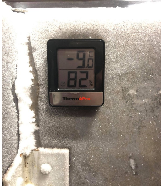
Figure 60. Access door temperature sensor
