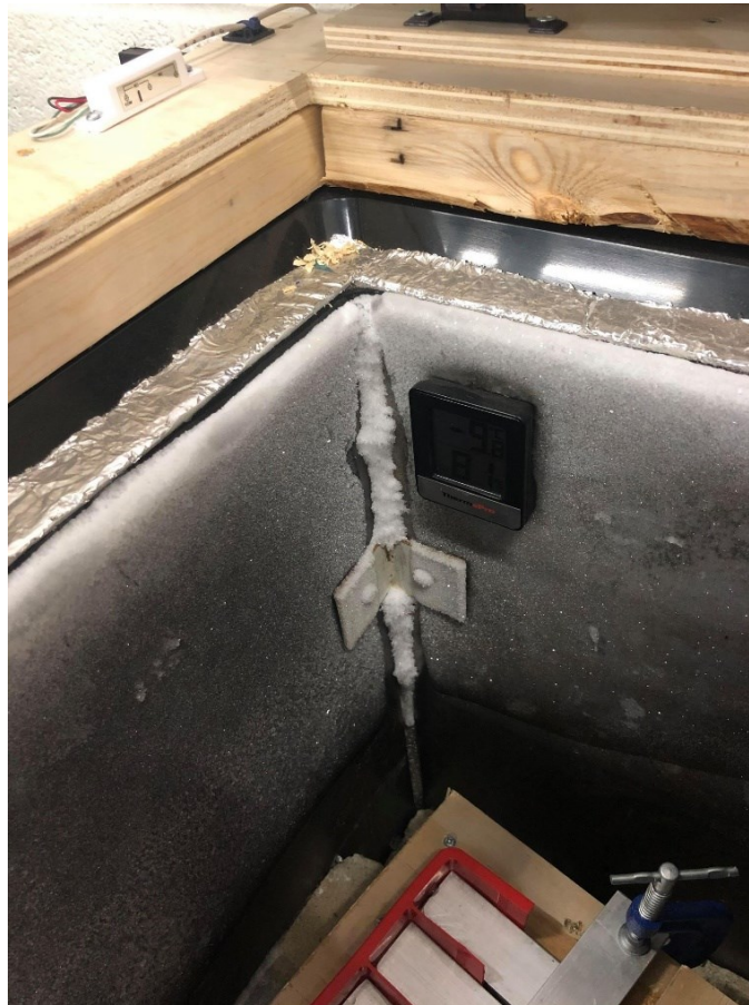
Figure 66. Steel plating inside CAT assembly
