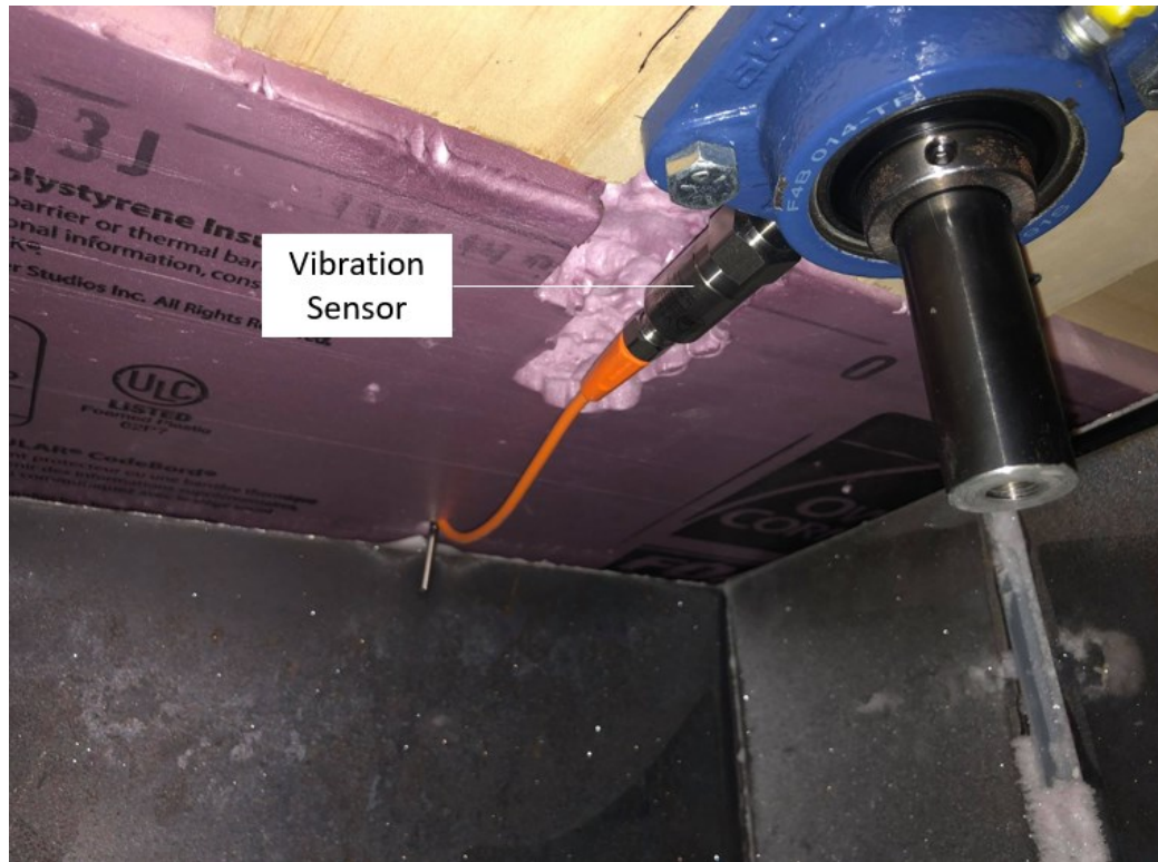
Figure 62. Vibration sensor mounted on the flanged bearing unit
