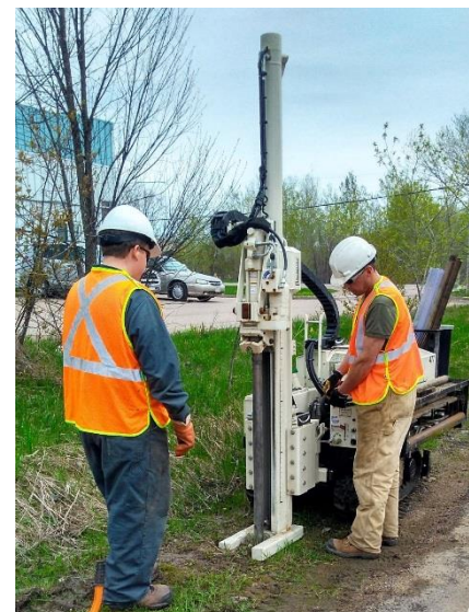
Figure 4: Push rig 54LT at core 1 sampling location (2017)
