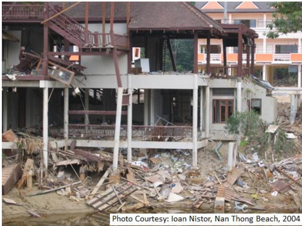
Figure 1-2 Destruction of the lower level of a resort building on the Nang Thong Beach, Thailand in 2004 (Nistor, 2011)
