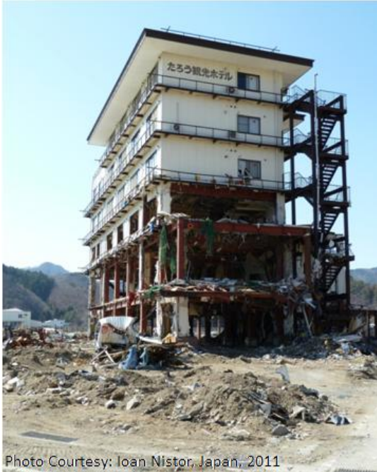
Figure 1-2 Hotel in Japan (Taro) with first three floors washed out by the 2011 Tohoku Tsunami (Nistor, 2011)
