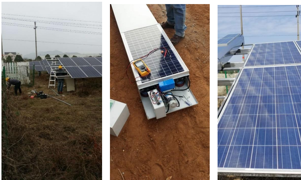
FIGURE 4.20 Photographs taken during the installation process of the robot.
