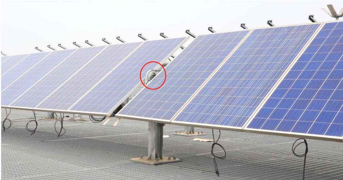
FIGURE 1.6 Bearing housing assembly at a solar electric power generation plant.
