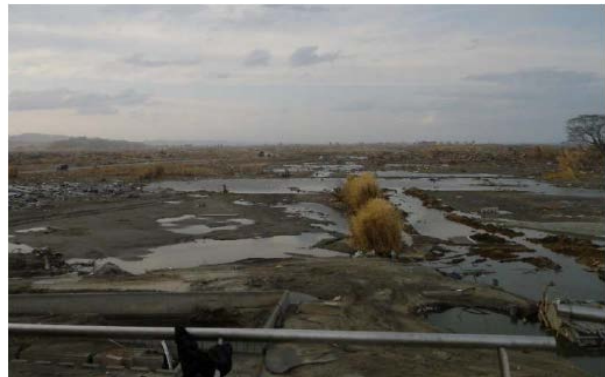
Figure 2-8: Overtopping scour, Taito Port, Japan. Case TO-1. Tonkin et al. (2013)
