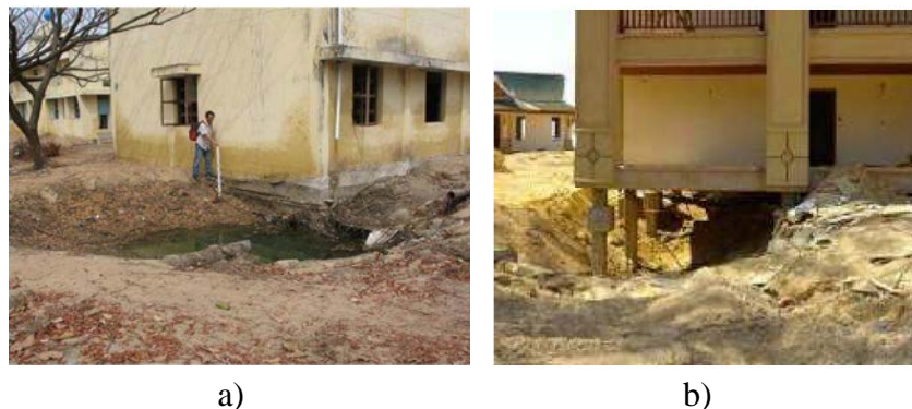
Figure 4-1: Typical tsunami-induced scour holes at building foundations: a) approximately 1.5 m deep in India, from the 2004 Indian Ocean tsunami (Yeh and Li 2008); b) Koh Khao, Thailand. Case SS-4 (Francis 2006)
