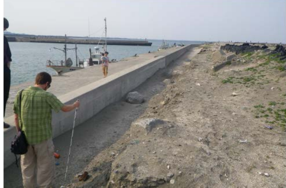
Figure 2-8: Overtopping scour, Taito Port, Japan. Case TO-1. Tonkin et al. (2013)
