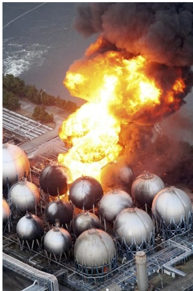
Figure 7: Fire in petroleum tanks following the 2011 Tohoku earthquake (Source: https://ehp.niehs.nih.gov/doi/10.1289/ehp.119-a290 )
