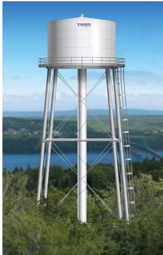
Figure 1: Municipal drinking water tank (Source: https://www.tankconnection.com/ask-the-expert/elevated-water-tanks )
