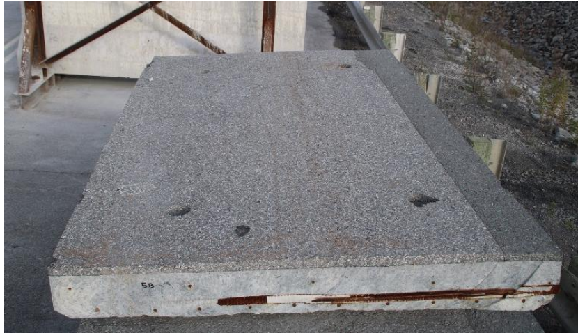
Figure 1-4 Infill slab extracted from Champlain Bridge
