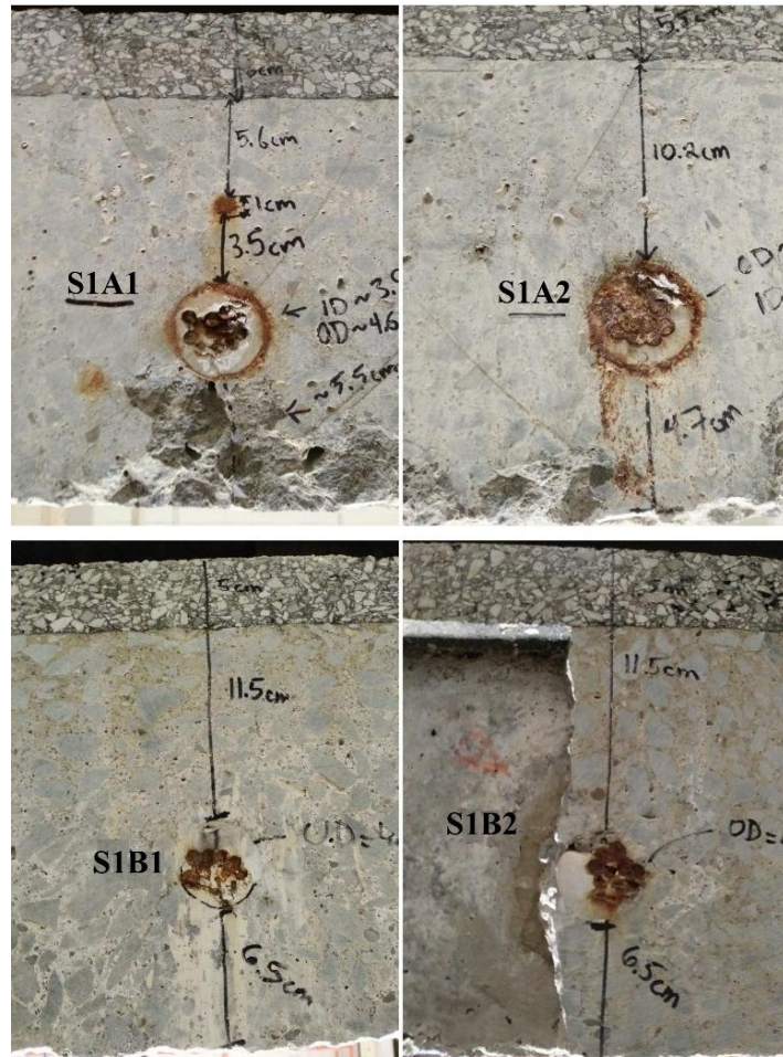
Figure 3-10. Tendon cross-sections at cut surfaces
