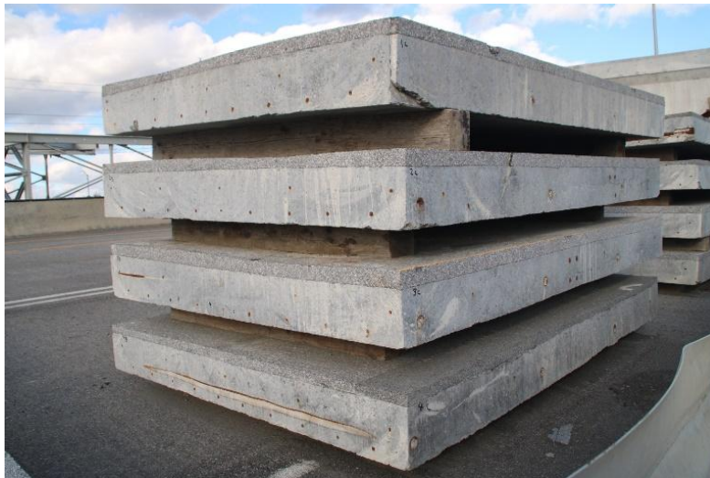
Figure 1-5 Infill slabs (stacked) extracted from Champlain Bridge
