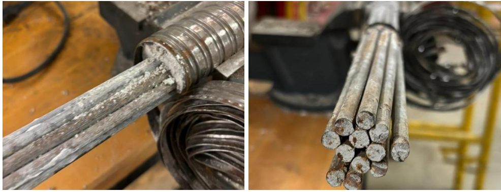
Figure 6-4 Extracted prestressing cables
