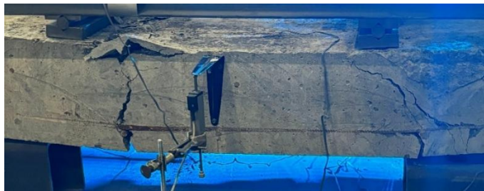
Figure 4-10 Flexural-shear failure observed in slabs (S7A3-S7B3)
