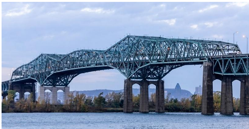
Figure 1-1 Former Champlain Bridge (reproduced from Jada, 2020)
