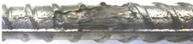
Figure 2-8 Typical pattern of pitting corrosion (reproduced from François et al., 2018)
