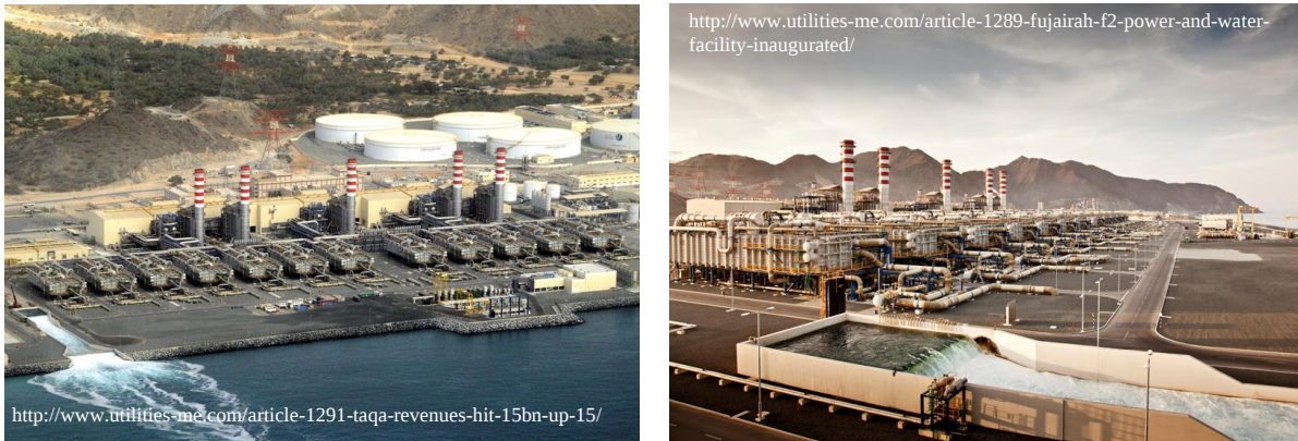
Figure 1.2 Fujairah power and desalination plant outfall discharging into Persian Gulf
