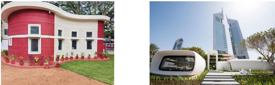
Figure 2-3: First 3D printed Post office in India (Left) and Dubai Future Foundation office (Right) (COBOD, 2023; Michelle Starr, 2016)
