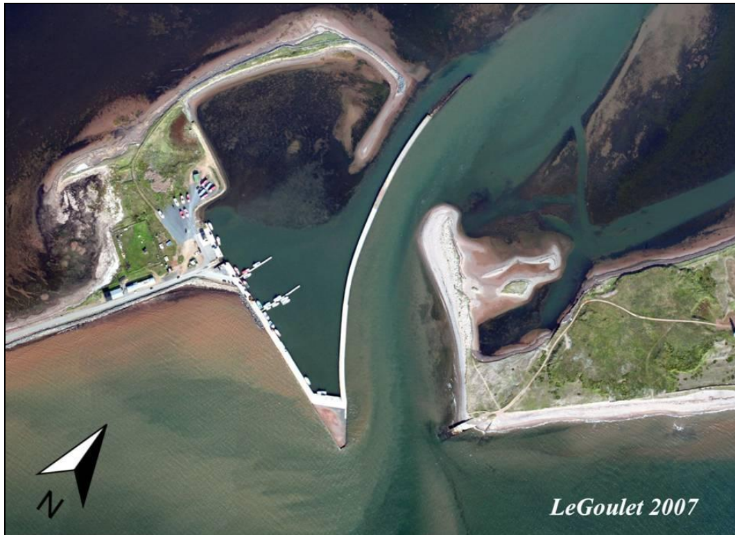
Figure 1.2: Aerial photograph of Shippagan Gully taken in 2007 (PWGSC, 2010).
