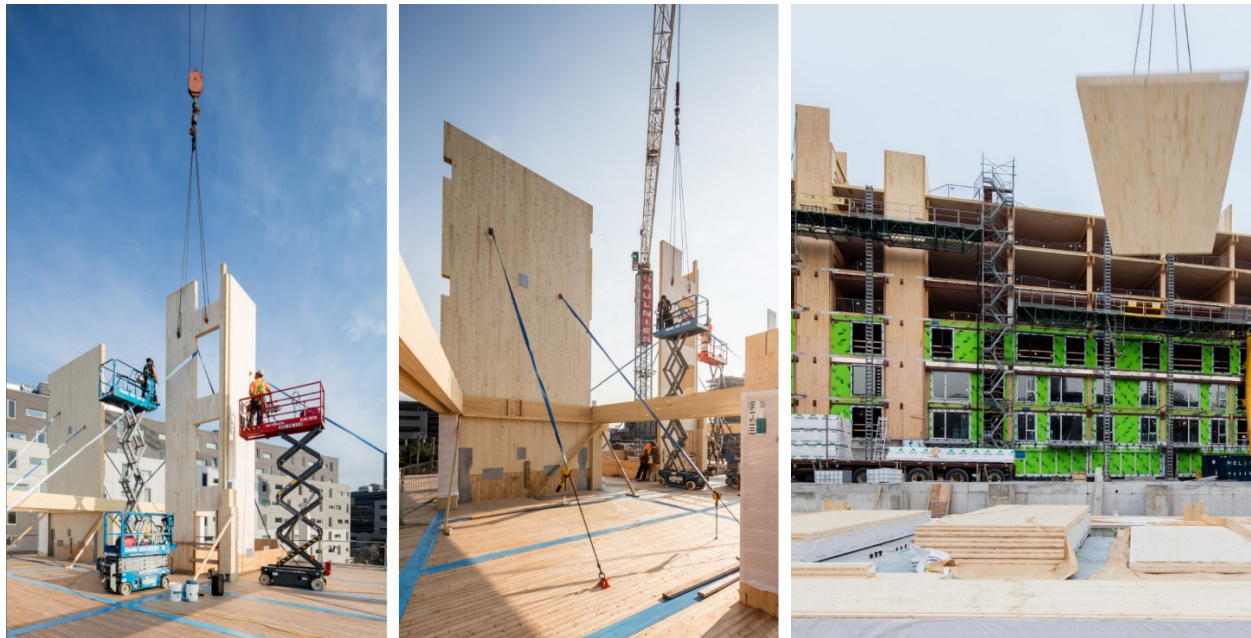
Figure 1.4: Another example of balloon-type construction: Photographs from the Arbora Condos project in Griffintown, Montreal. (photographed by Adrien Williams 2 ; source: https://www.nordic.ca/en/projects/structures/arbora )
