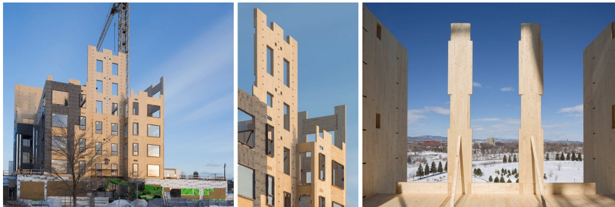
Figure 1.2: Example of balloon-type construction: Photographs from the 13-storey Origine building in Quebec City, Canada (2018) (photographed by Stéphane Groleau 1 ; source: https://www.nordic.ca/en/projects/structures/origine ).
