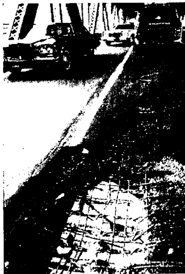
Figure 1.2 – Exposed Rebar [2]
