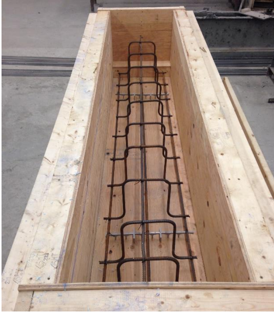
i) Construction of formwork and installation of reinforcement
