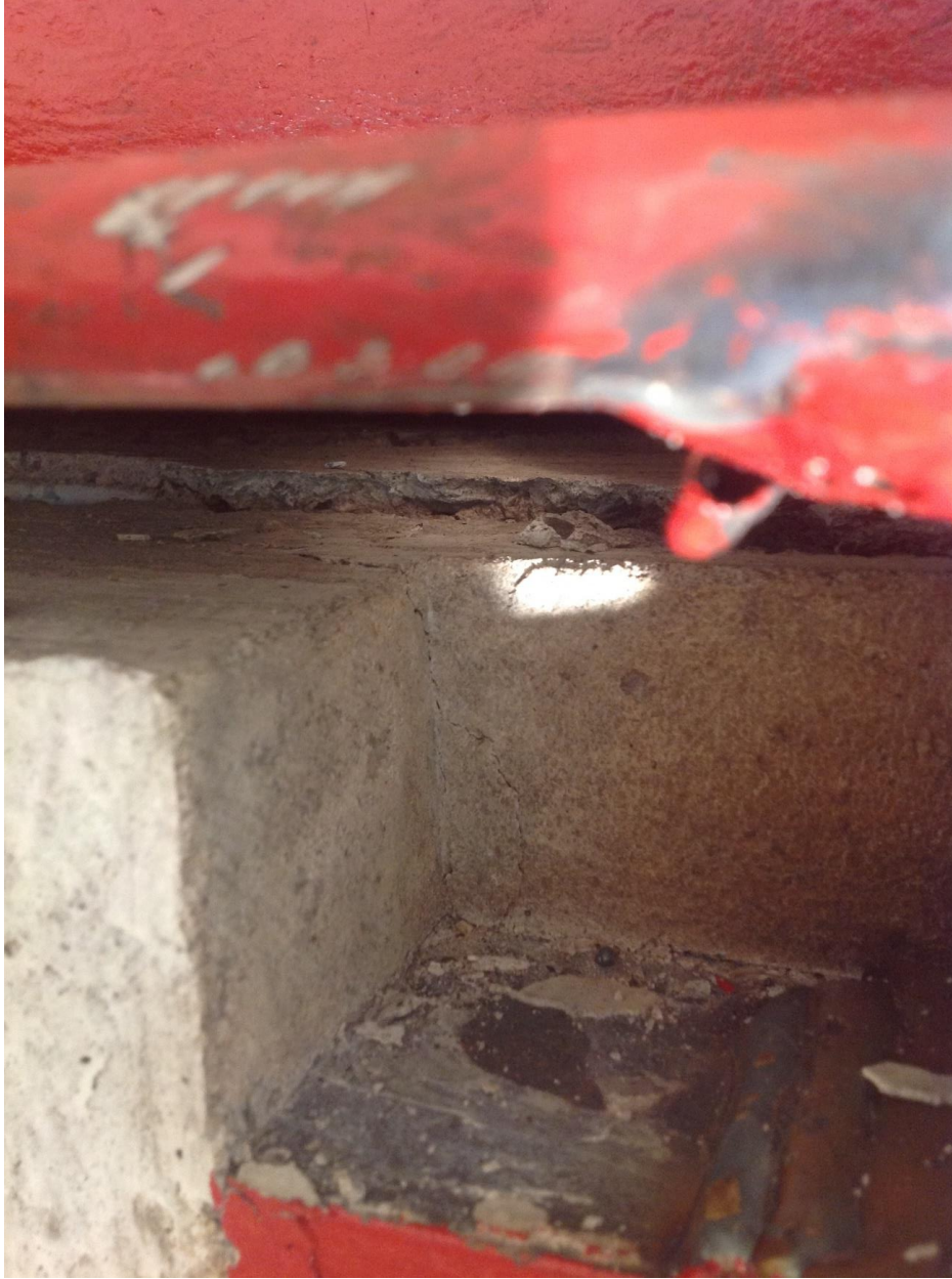
Figure 4.27 – NCTS-M: Typical Crack Development near Upper Supports during Test 1
