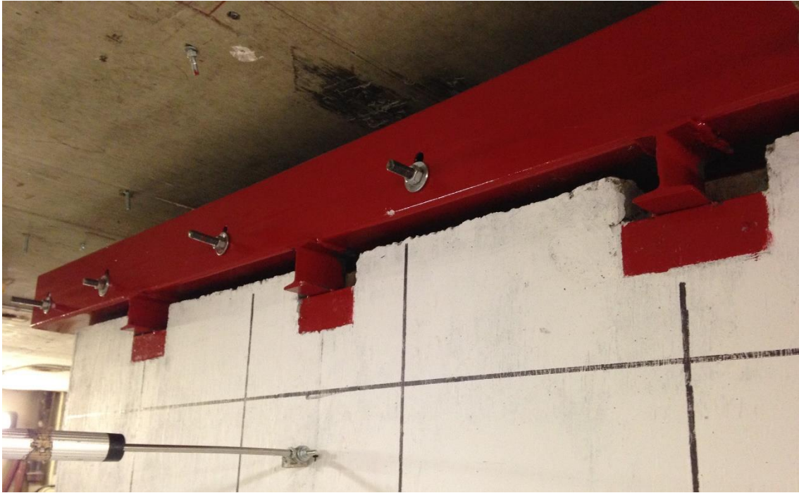
Figure 3.23 – Close-Up of Upper Support System
