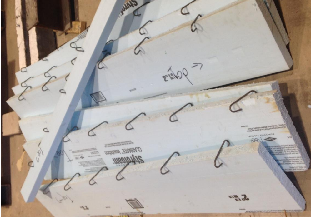
Figure 3.6 – Typical Installation of Shear Ties Prior to Casting
