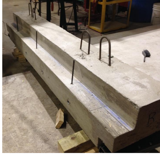
ii) Completed base support with dowels and panel layout marking
