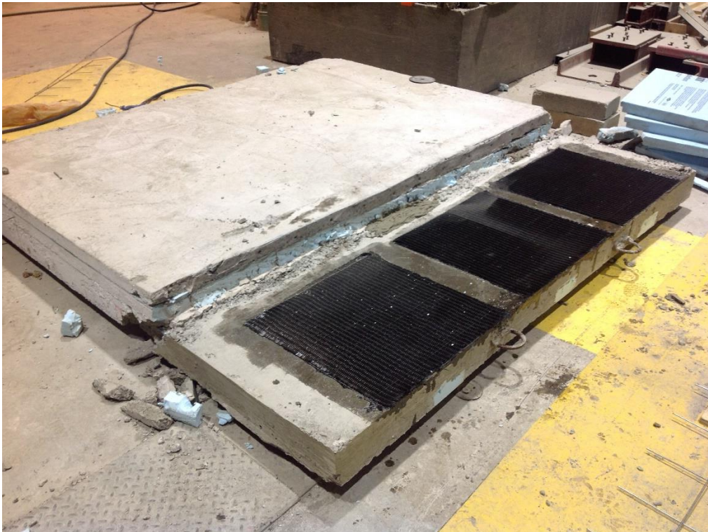
Figure 3.10 – FRP Support Retrofit Installed Prior to Casting of Architectural Face
