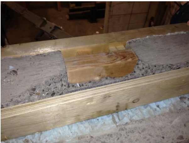
ii) Installation of formwork
