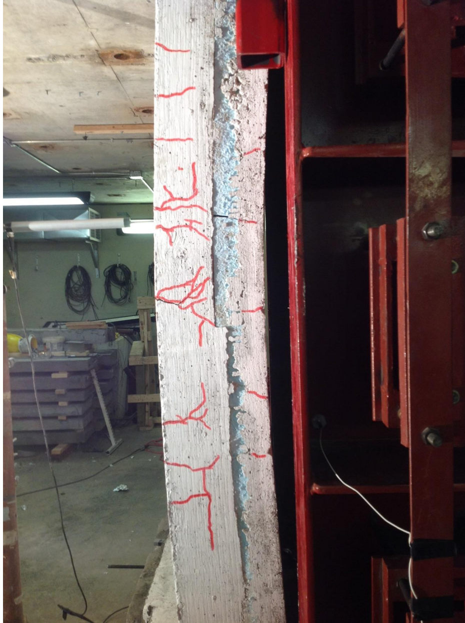
Figure 4.23 – NCTS-M: Side View with Flexural Cracks (Test 3)
