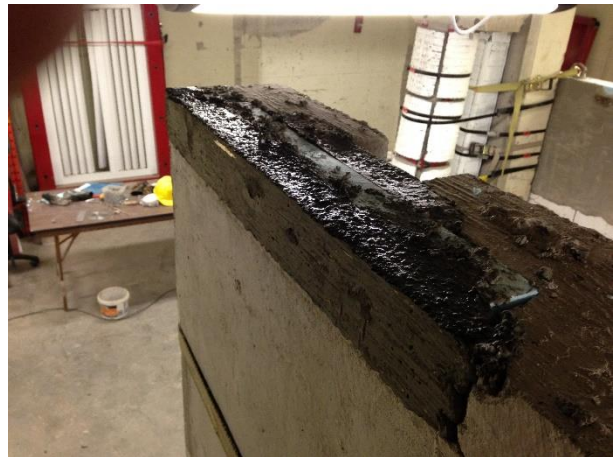
iii) Recasting concrete into the damaged area
