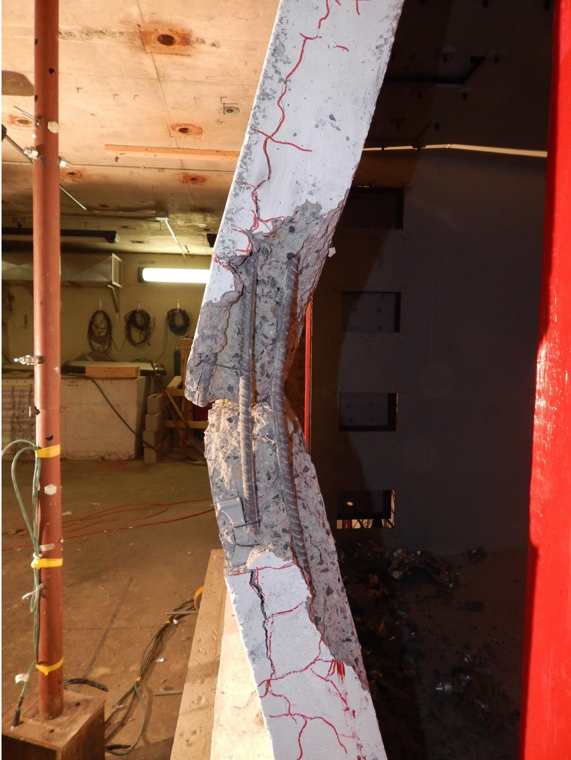
Figure 4.2 – SRC-1: Side View at Conclusion of Testing (Test 5)
