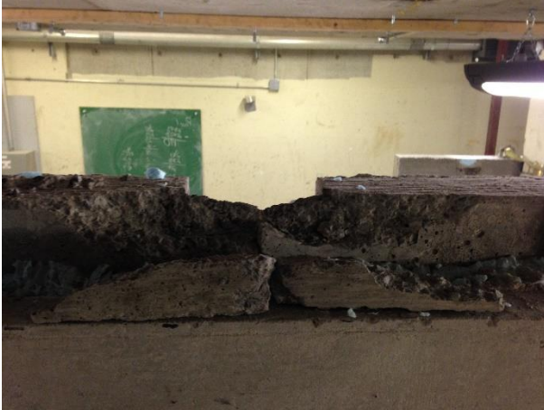
i) Upper Connection-3 Inspection and removal of concrete near damaged connections
