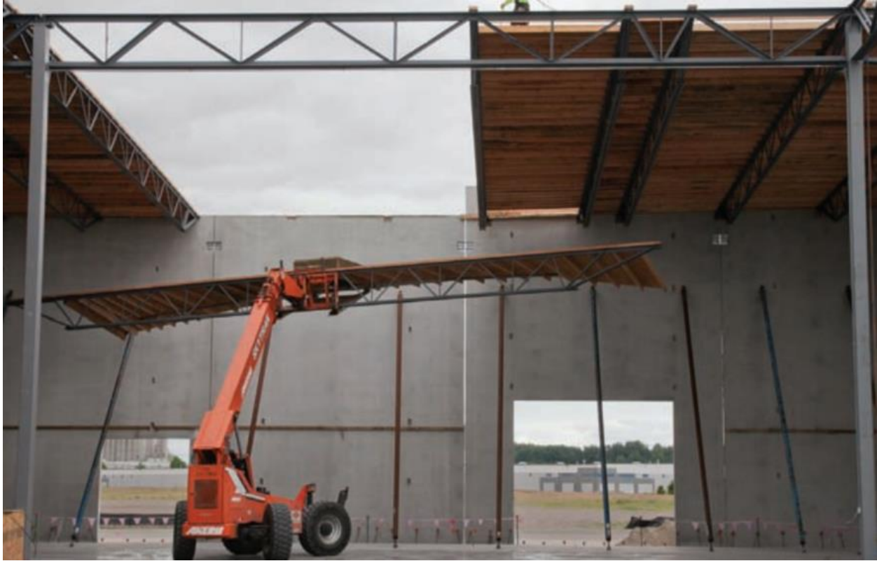
Figure 1.1 – Tilt-Up Panels used in Practice (Panel-to-Frame Upper Connections)
