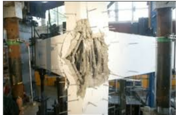
f) Beam-column joint failure (Ref 6.)
