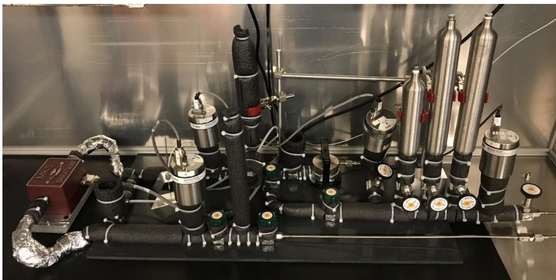
Figure 2.2 The picture of the inside of the controlled temperature chamber. Referring to Figure 2.1, the components on the picture's left and right are DPT1 and APT3, respectively.
