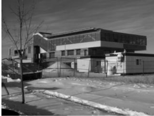
Fig. 4.2. Mosaic Centre, Edmonton, Alberta
