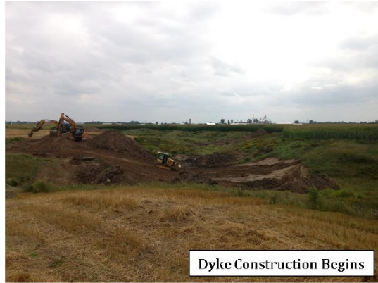
Trenching to Key In Dyke
